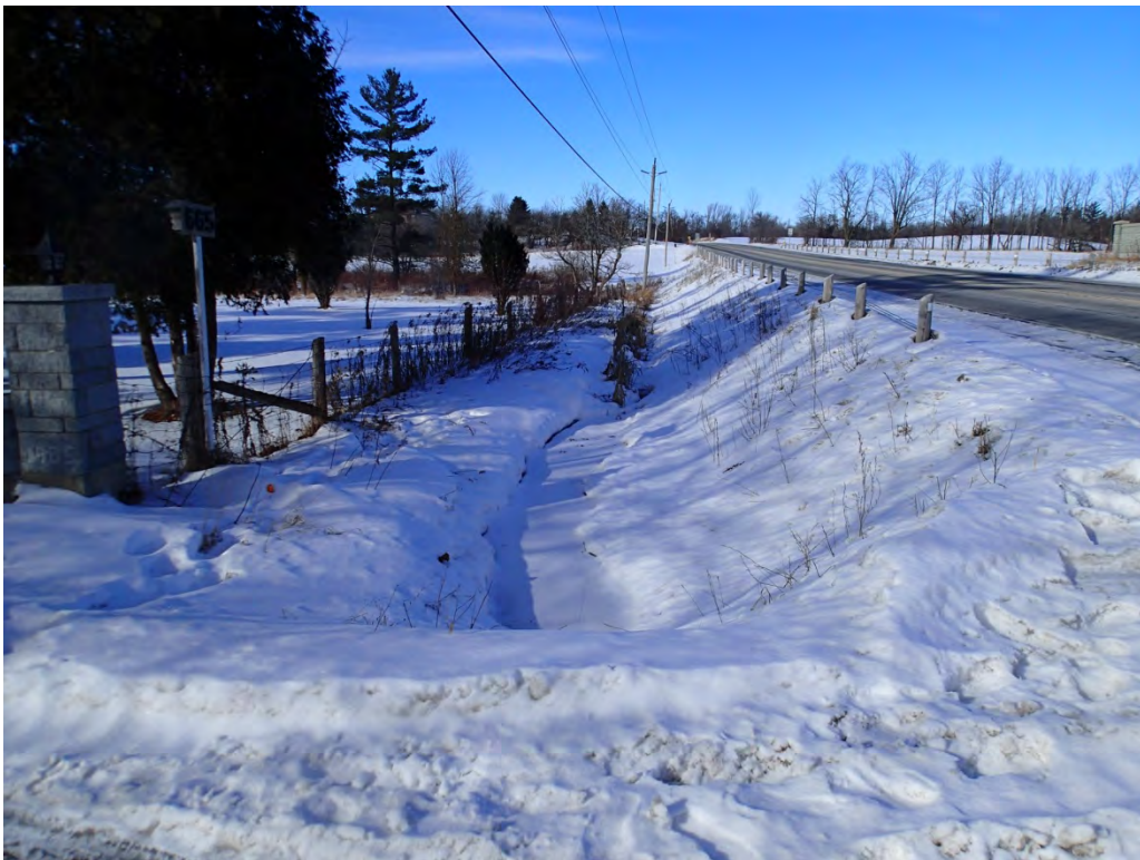
Photo 16: 16 Habitat reach WT1 downstream from driveway culvert. January 2015.
