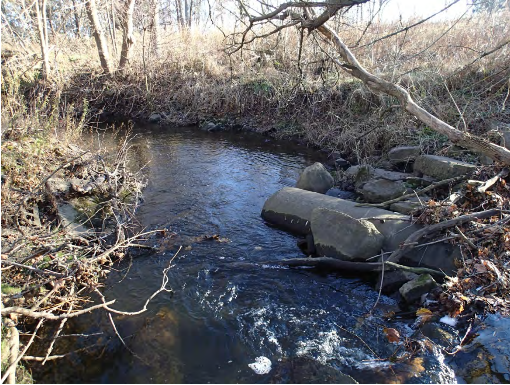
Photo 5: Abandoned crossing in Reach L4. November, 2013.
