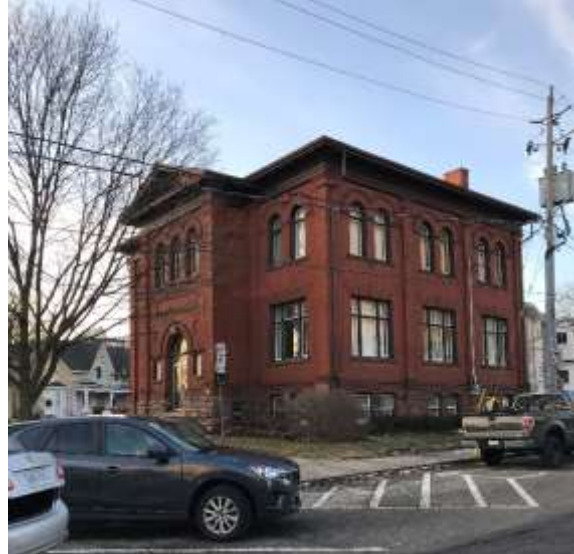
Photo 2: View of Carnegie Library (City owned building) on west side of Dorset Street
