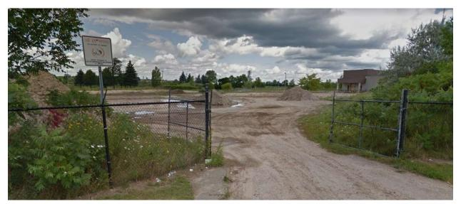
**Figure 2:** Existing City of Waterloo Snow Storage Facility from Frobisher Drive. Facility design features include chain link fencing with barbed wire as well as perimeter grading along the east and north to mitigate drainage impacts to neighbouring properties. This a Google Street View photo from August 2015. Note the mud and sediment accumulation that remains well into the summer.
