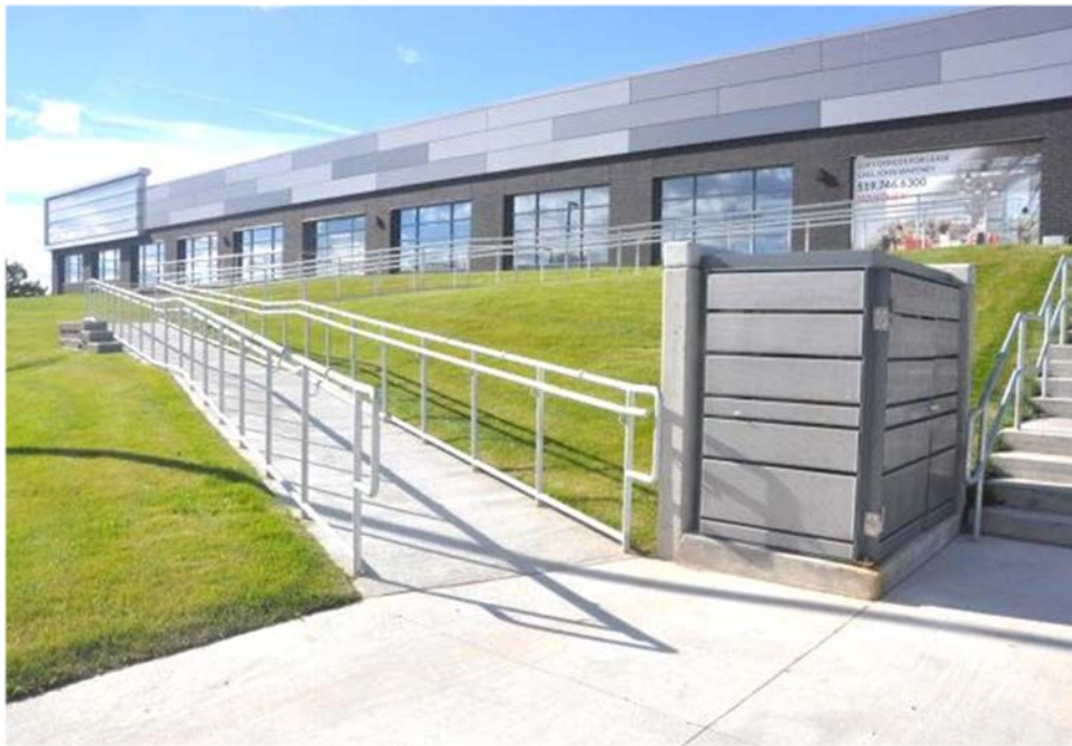
Figure 14: Example of a ramp with appropriate handrails and slope levels
