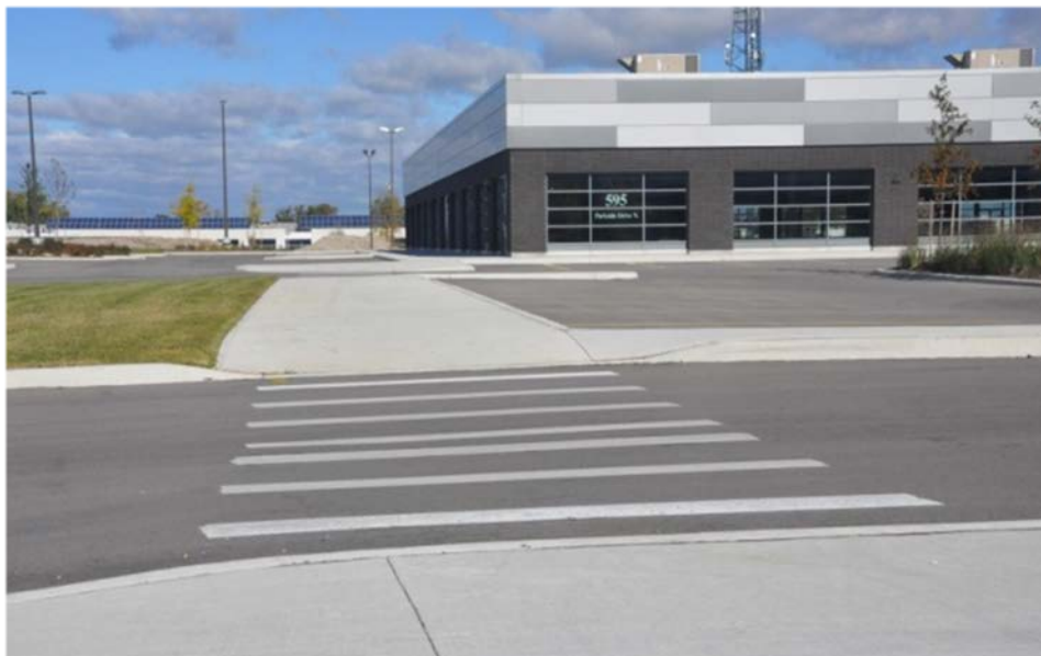
Figure 18: Example of a curb ramp located at a cross-walk
