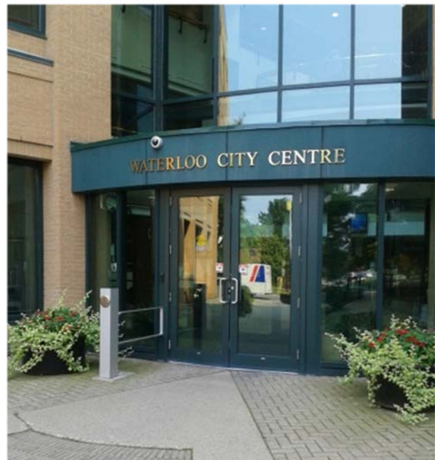
Figure 28: Example of an automatic swing door with a bollard mounted push plate and guard rail
