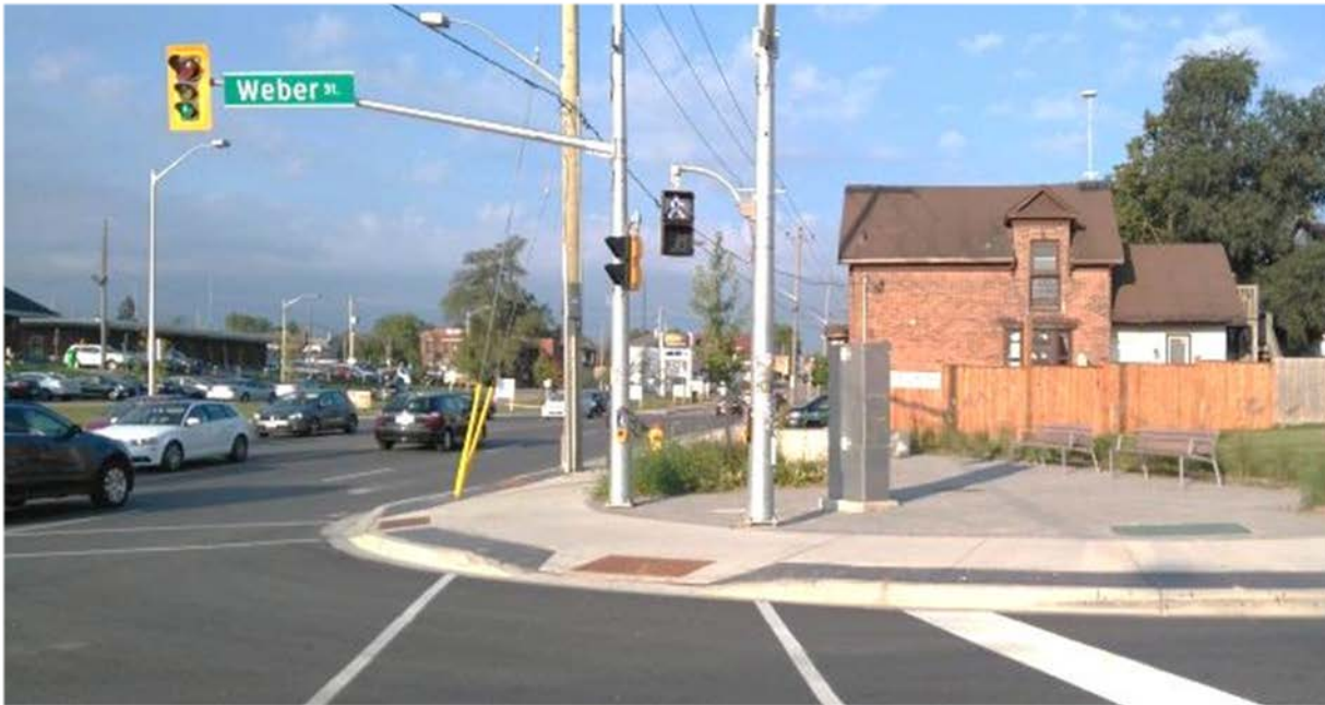
Figure 12: Drop curb with tactile surfacing located at an intersection
