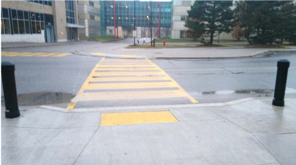
Figure 19: Example of a tactile warning surface
