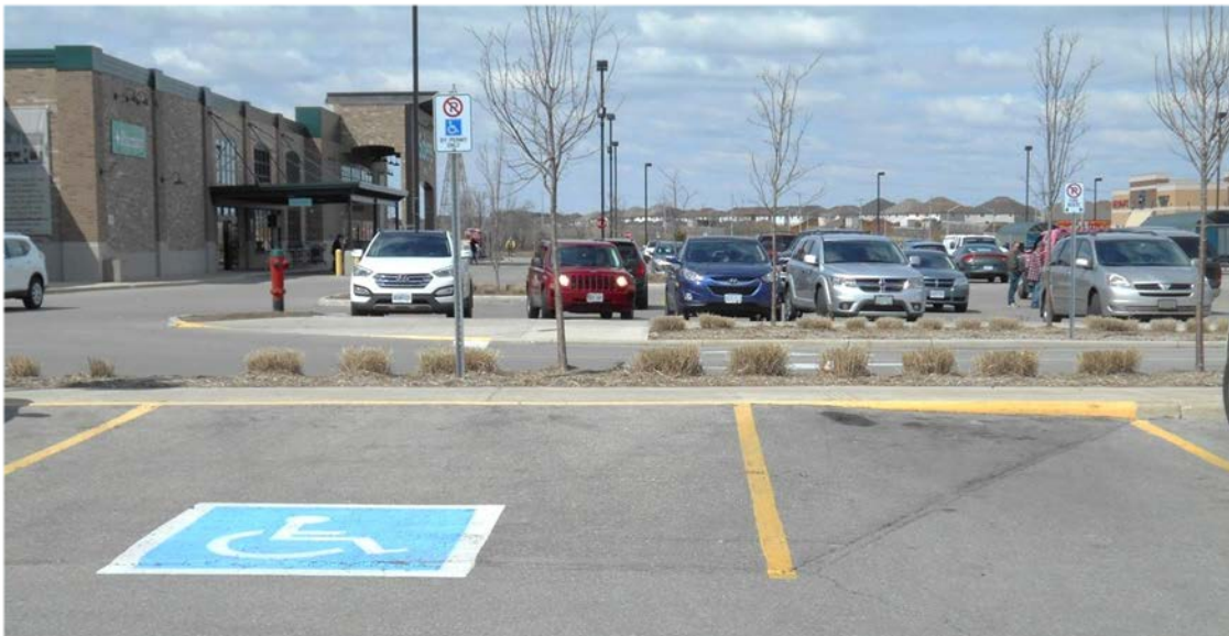
Figure 4I: Example of benched asphalt flush with curb along accessible parking spaces
