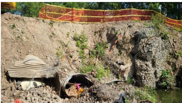
Pedestrian Bridge Bank – Emergency Repair
