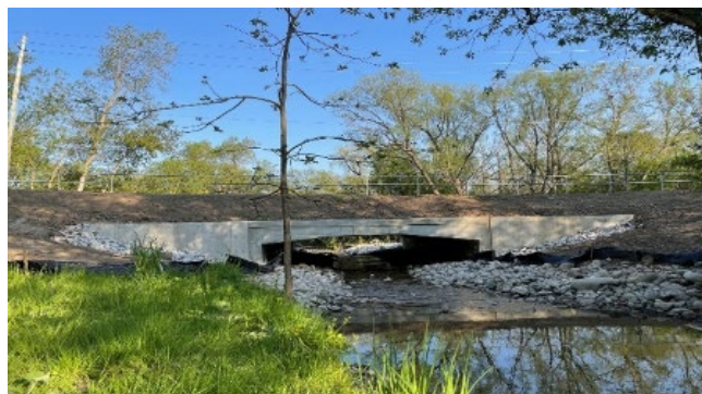
New Pedestrian Bridge
