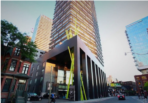
Image 53: 125 Peter Street in Toronto The podium base prevents strong winds at street level and provides a colonnade to create a cover space that is comfortable even in the rain.
