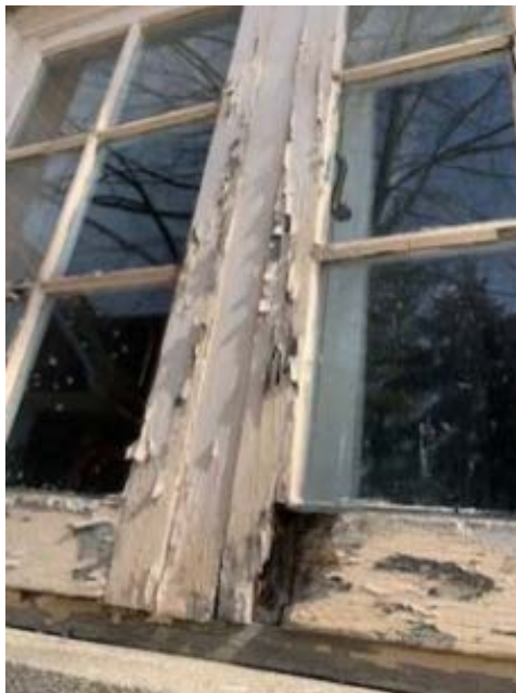
Figure 3: Existing South Façade (Rear) Window – Existing windows (excluding front façade) to be replaced with vinyl windows.
