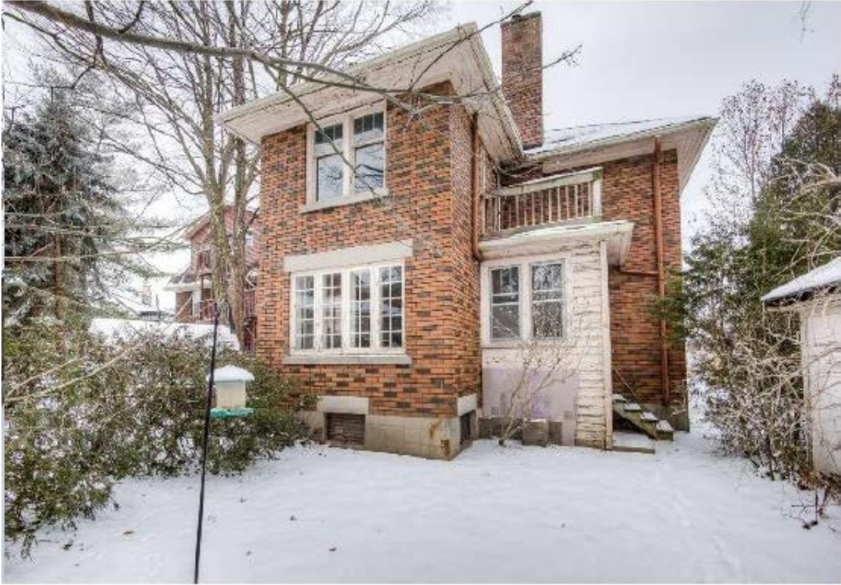
Figure 2: Existing South Façade (Rear) – Existing addition with porch to be demolished and replaced with a two (2) storey addition.
