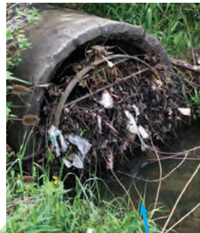
9. Debris in Trash Racks
