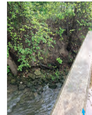
1. Eroded Outfall
