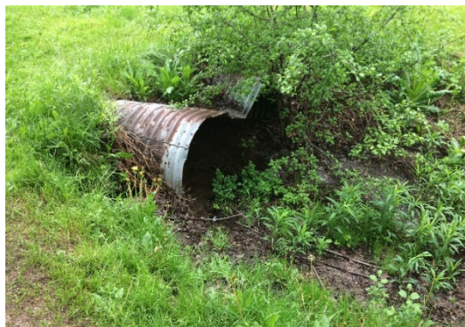
Photo 18 Overflow culverts near historic dam
