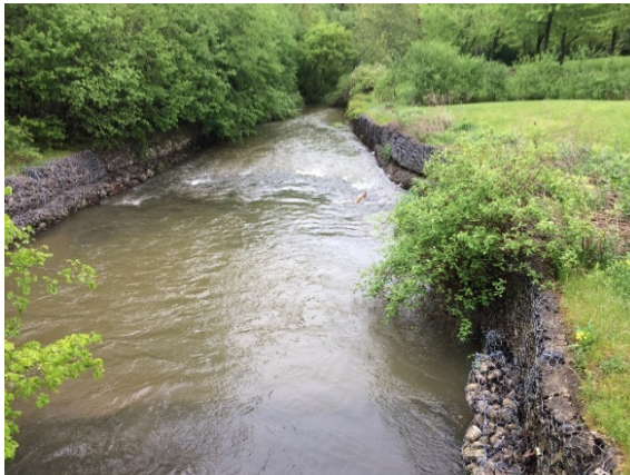
Photo 16 Undermined gabions.
