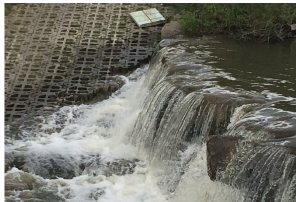
Photo 30. Terrafix access road at outlet structure.
