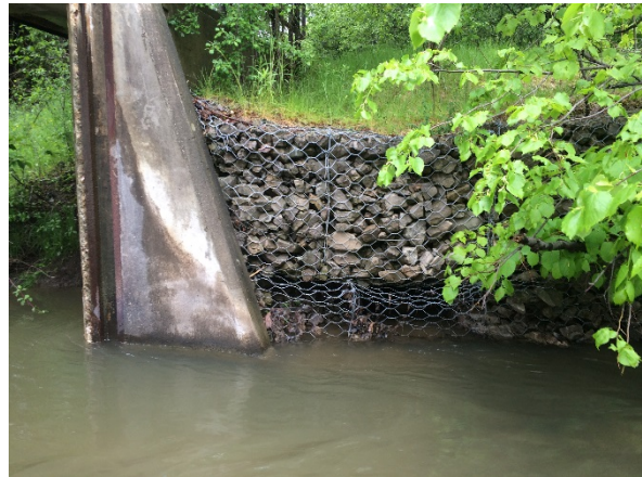
Photo 4. Failing gabions at historic dam
