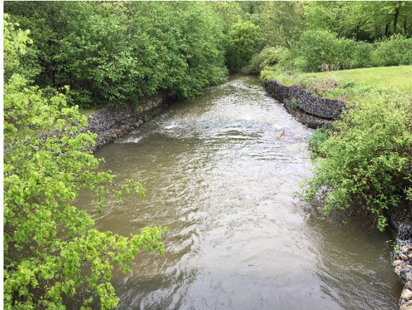
Photo 3. Gabions downstream of historic dam.
