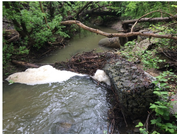
Photo 1. Eroded bank, Clair Creek at Westmount Rd. N.
