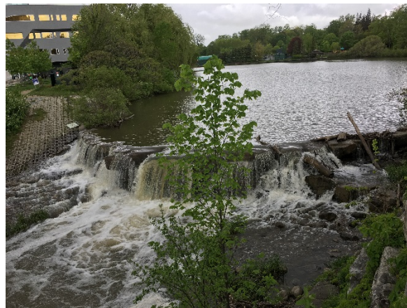
Photo 12. Armourstone outlet structure, Silver Lake.
