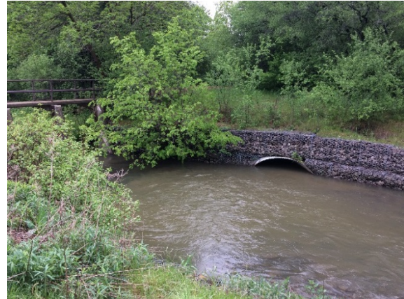
Photo 17. Undermined gabions.
