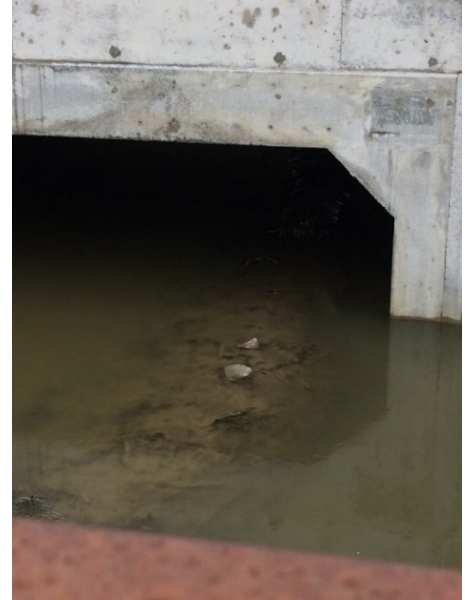
Photo 21. Sediment deposition in Silver Lake, downstream of LRT tracks.
