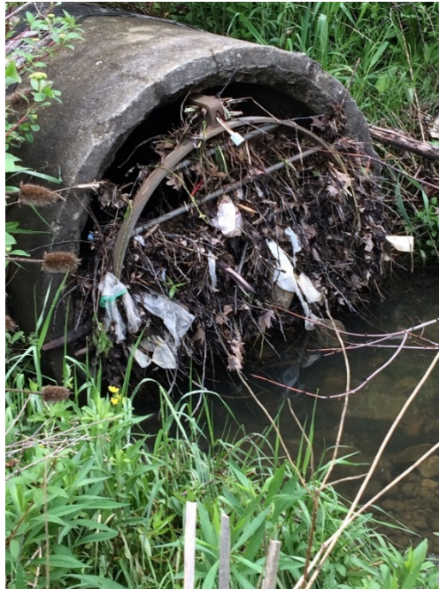
Photo 28. Debris in trash rack of stormwater outlet.
