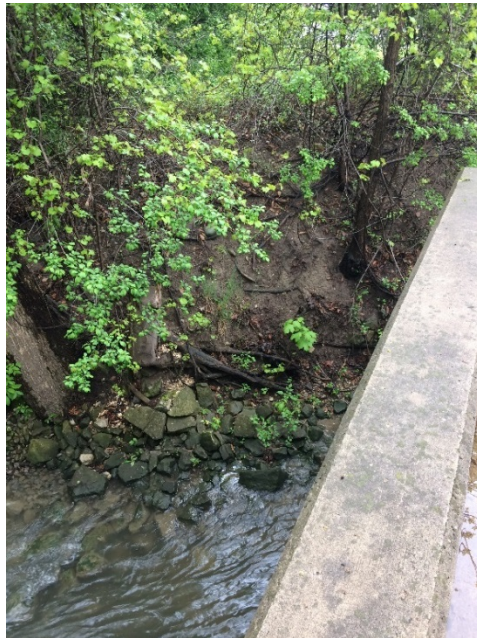
Photo 13. Bank erosion at Laurel Creek at University Avenue.
