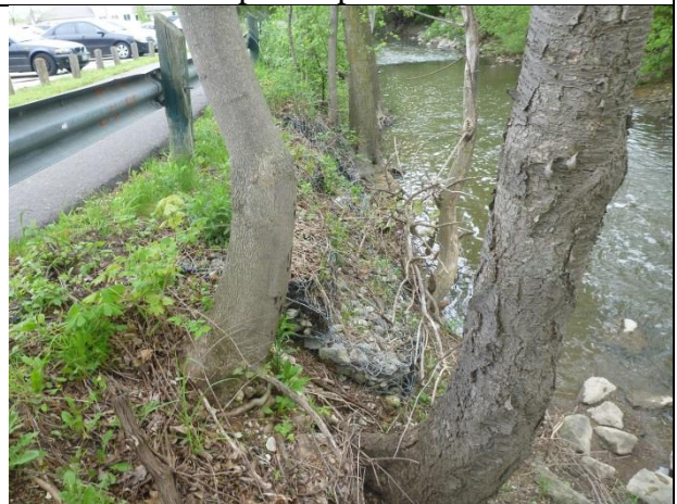
Failing gabions on slope adjacent to trail
