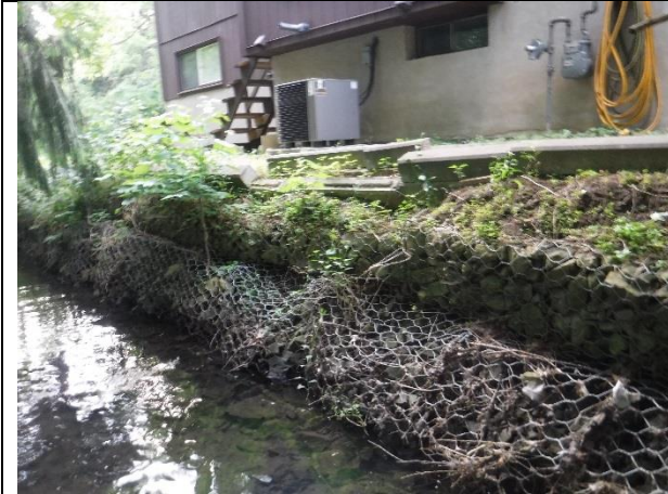
Failing gabion baskets
