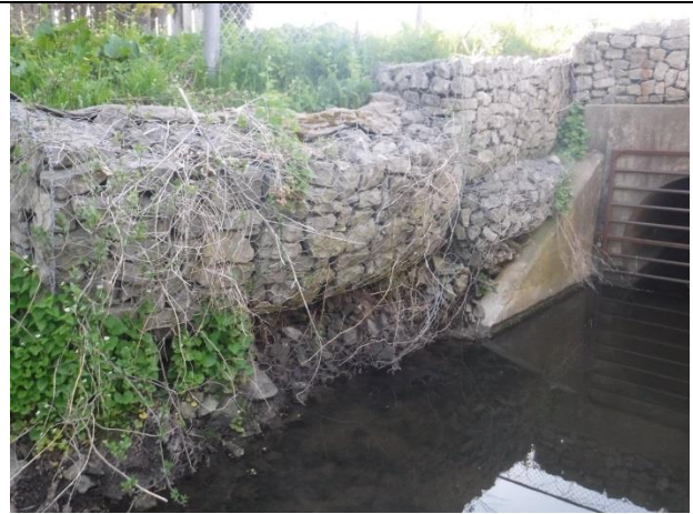
Condition of gabion baskets on left bank
