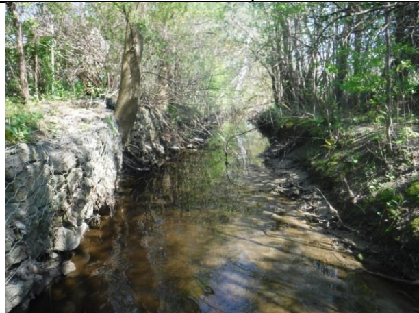
Location 2 – Failing gabion basket treatment on left bank
