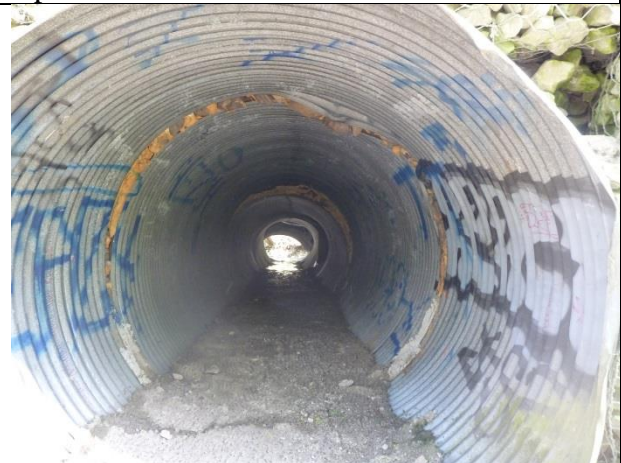
Shearing at joints in culvert
