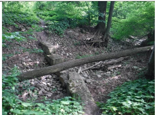
Armourstone weirs downstream of stormwater management facility outfalls
