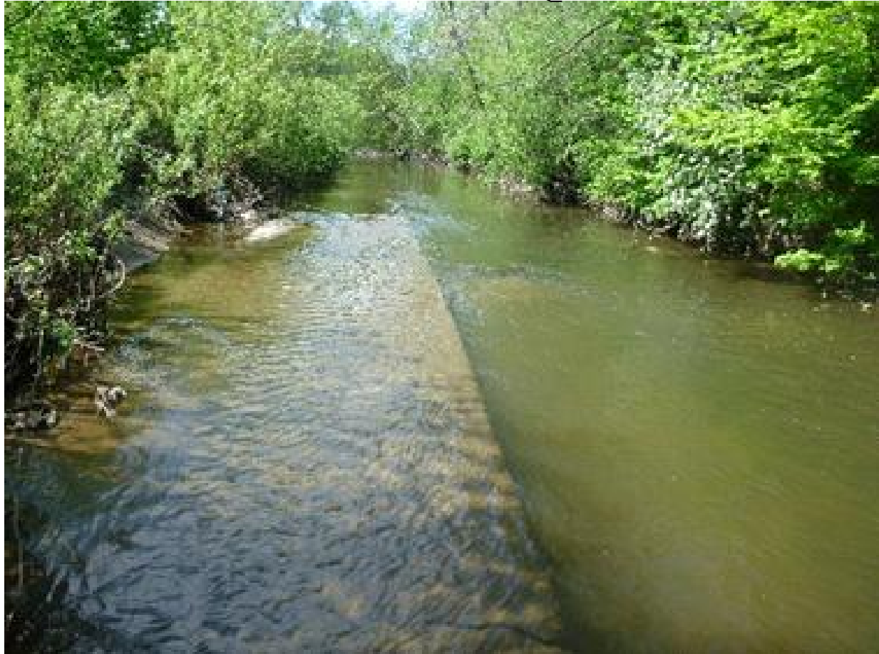
EXPOSED CONCRETE ON CHANNEL BED
