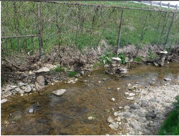
Undermining of fence posts
