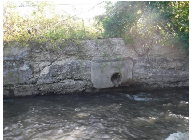
Storm sewer outfall in concrete wall
