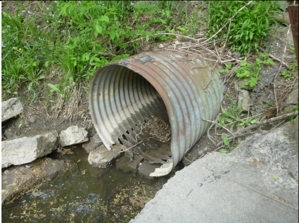
Storm sewer outfall in poor condition
