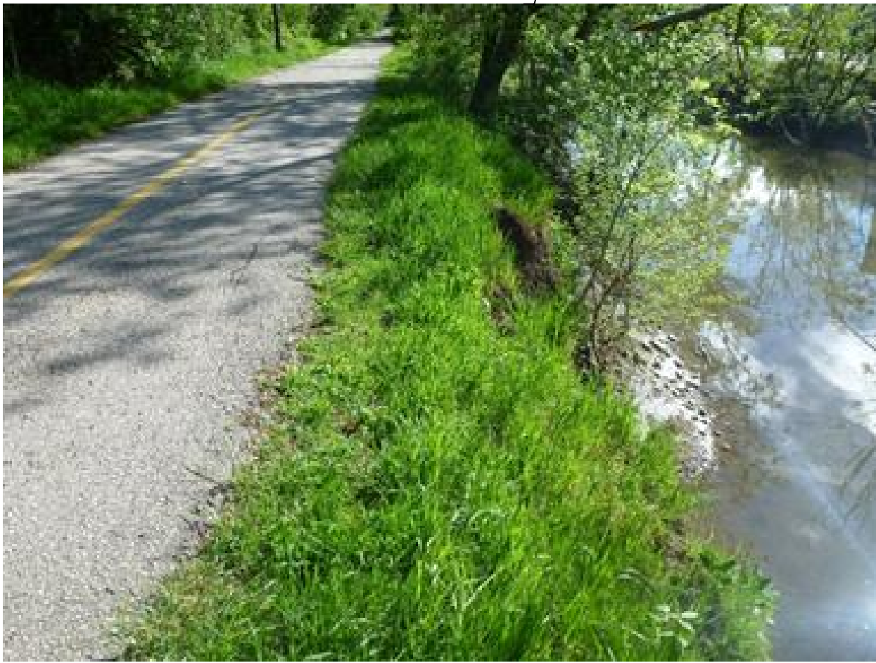
NEAR VERTICAL BANK EROSION PUTTING TRAIL AT RISK
