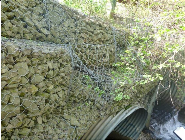
Failing gabion baskets
