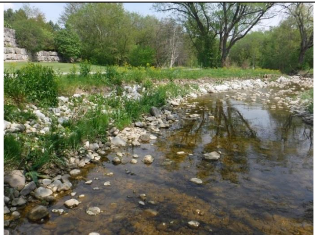
Roundstone bank treatment is slumping and vegetation on bank is primarily herbaceous
