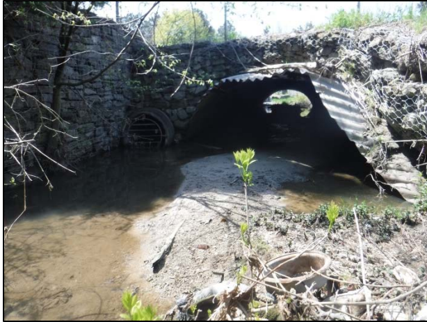
Figure 8-6: Downstream end of failing culvert under Albert Street at CDR-E3
