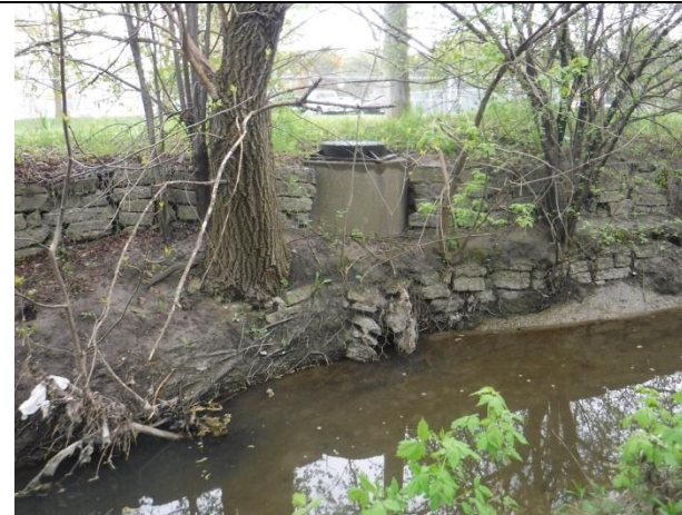
MH behind failing gabion basket treatment
