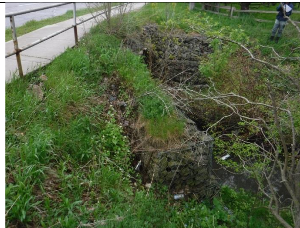
Outflanked gabion basket headwall
