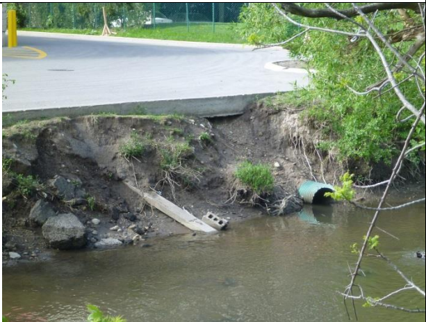
Undermining of loading area pavement
