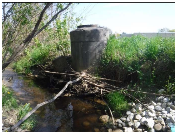
Figure 8-2: Sanitary maintenance hole in creek at CDR-E4
