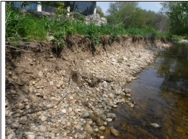
Roundstone is failing and bank is near vertical and eroding towards the path
