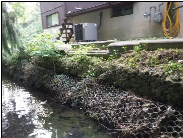
Figure 8-7: Failing gabion baskets with building located within 5 m of the top of bank at CLR-T1-E1
