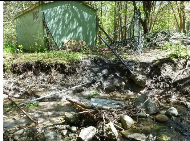
Undermined and leaning fence post
