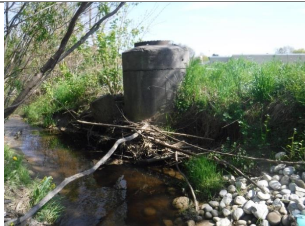
Location 1 – Scoured bank immediately upstream of MH
