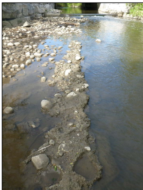
Figure 8-3: Exposed concrete on channel bed at LRL-E6
