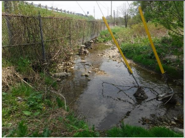
Guy wires in channel. Sanitary sewer crosses under creek.
