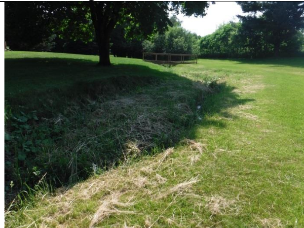
Manicured lawn to top of bank with bank slumping and eroding
