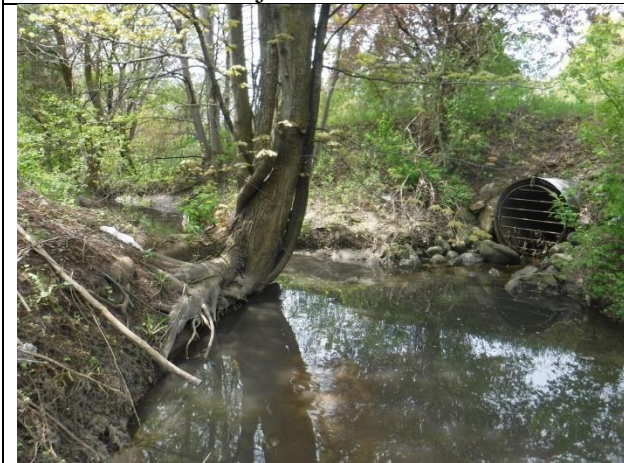
Storm sewer outfall and tree deflecting flow to opposite bank
