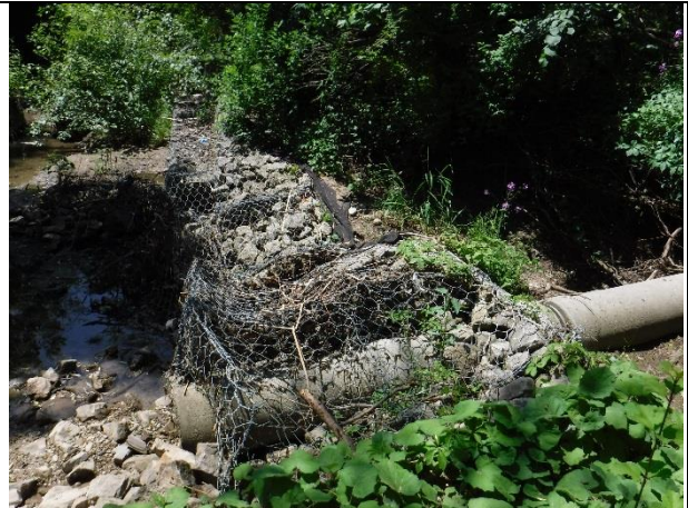
Failed gabions over storm sewer outfall
