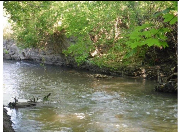
Outflanked downstream end of leaning concrete wall
