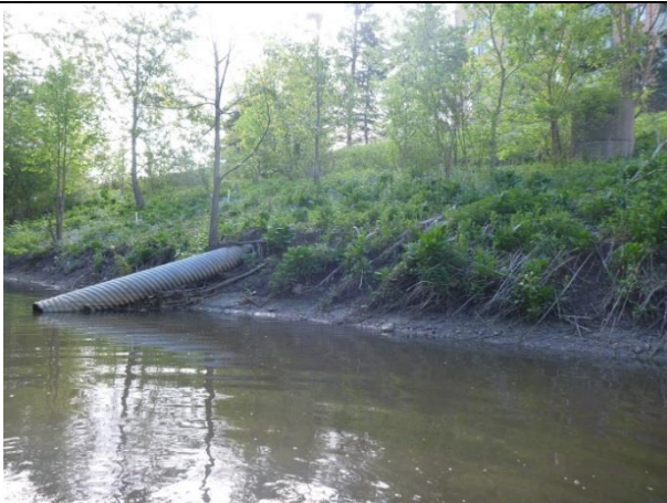
Near vertical bank erosion in front of MH. Failing private outfall.
