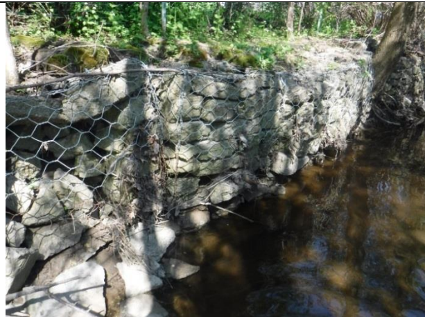
Location 2 – Emptying gabion baskets
