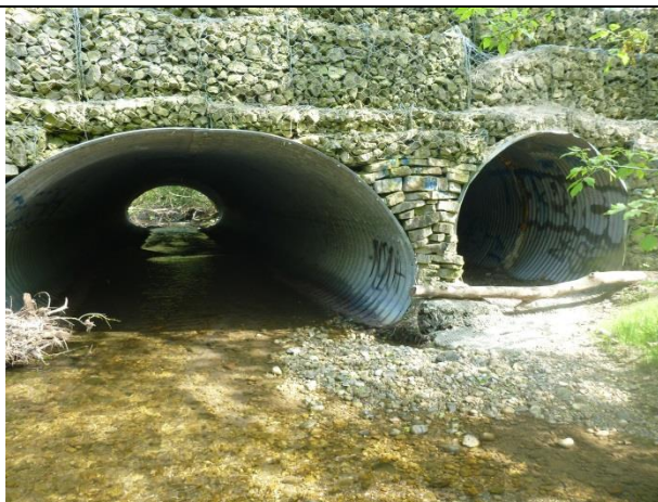
Upstream face of culverts
