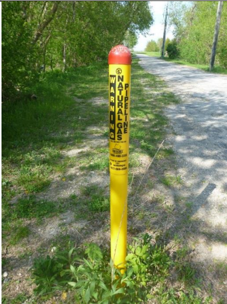
Marker for natural gas pipeline crossing creek
