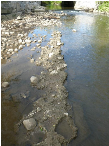
Exposed concrete on bed
