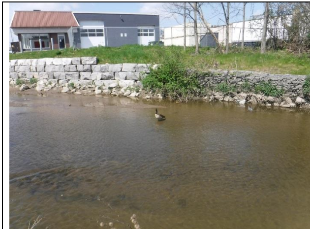
Failing gabions at end of armourstone wall
