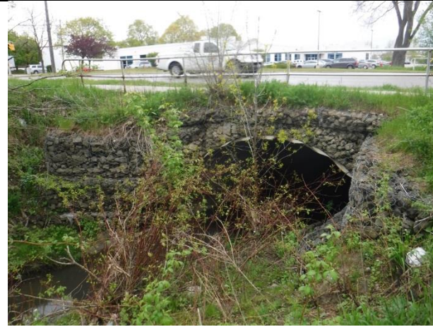
Failing headwall on upstream side of Weber Street
