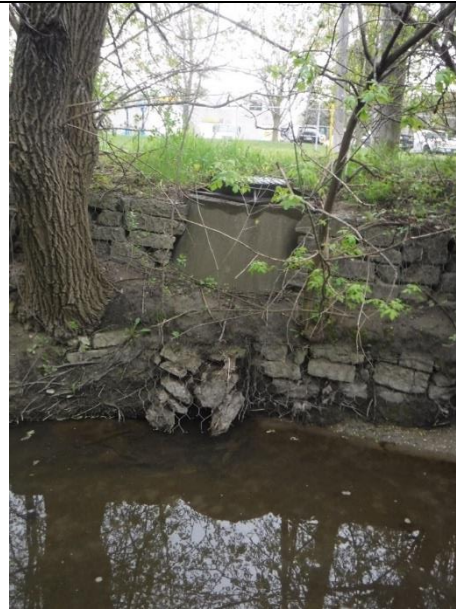
MH behind failing gabion basket treatment
