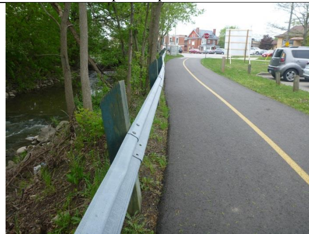
Top of eroding bank in close proximity to trail
