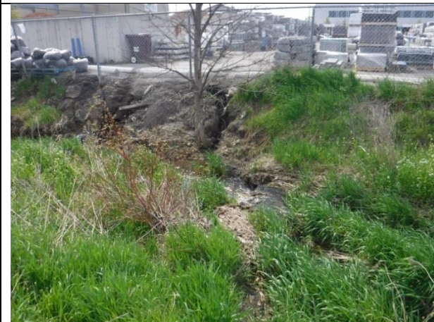
Undermining of fence where storage area runoff enters the creek
