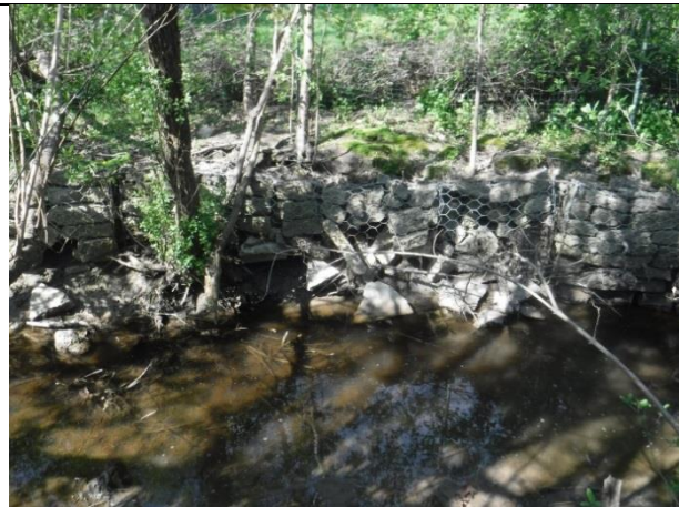
Location 2 – Failing gabion baskets on left bank
