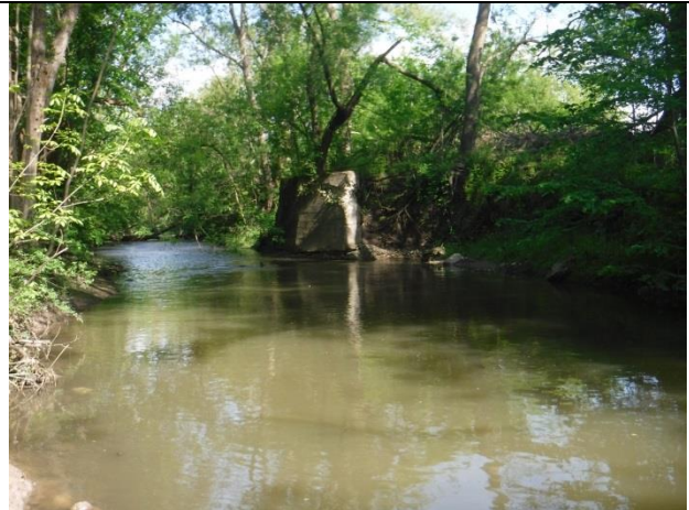
Outflanked old concrete abutment
