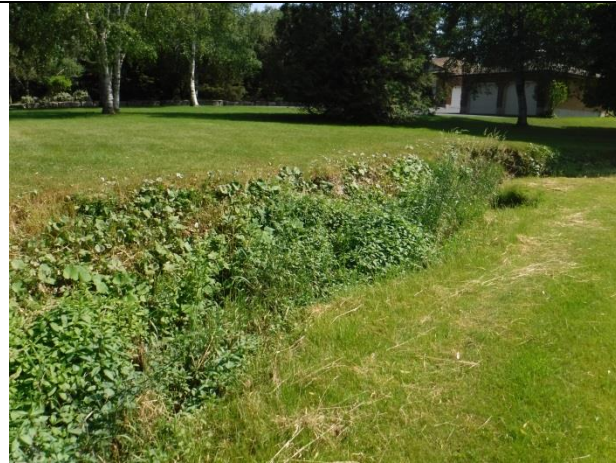
Manicured lawn to top of bank with bank erosion throughout channel
