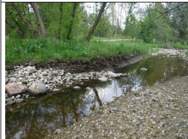
Slumping roundstone with eroding bank downstream
