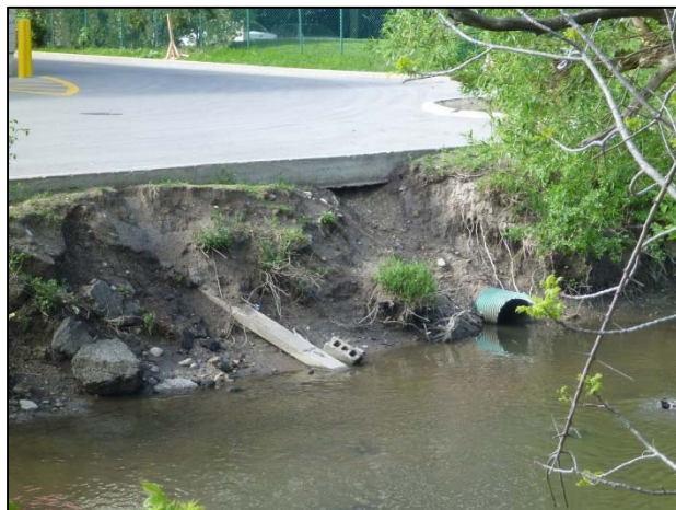
Figure 8-5: Undermining of paved loading area on private property at LRL-E7
