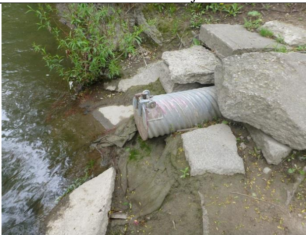
Existing treatment around storm outfall
