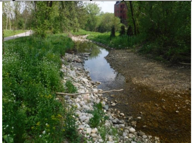
Roundstone treatment with herbaceous vegetation on bank
