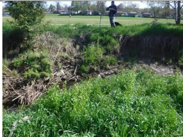
Location 3 – Bank erosion towards sanitary sewer MH
