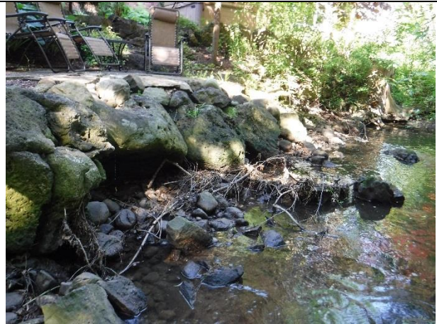
Failing boulder bank treatment
