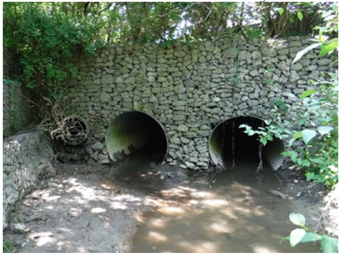
GABION BASKET HEADWALL AT COLUMBIA STREET WITH LOWER BASKETS EMPTYING
