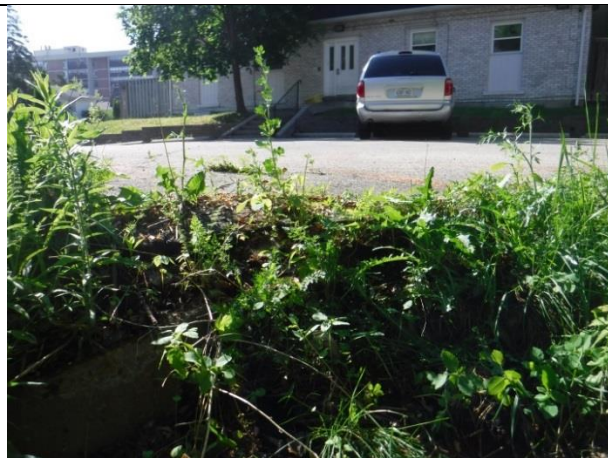
Bank erosion adjacent to parking lot with top of bank and exposed MH in foreground
