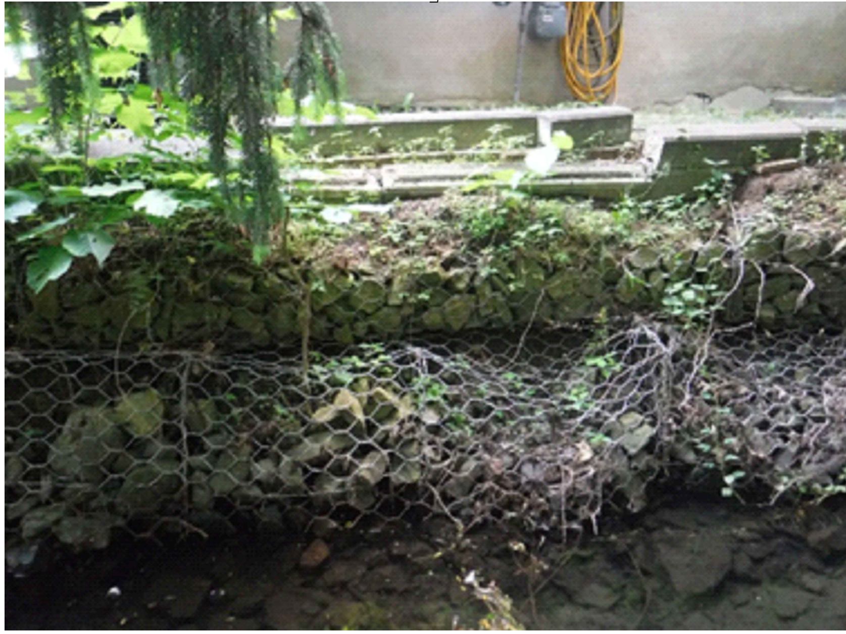
FAILING GABION BASKETS
