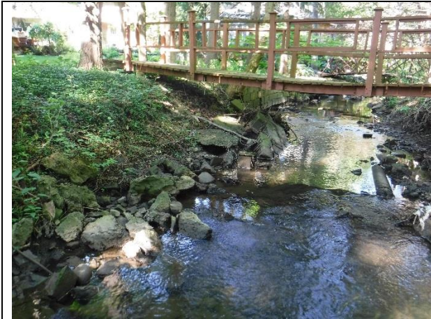
Pedestrian bridge and failing concrete block bank treatment
