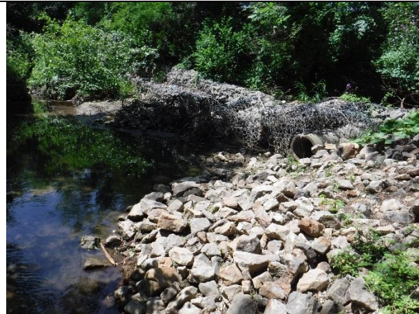
Rip rap with failed gabion baskets and storm outfall in backgrounds
