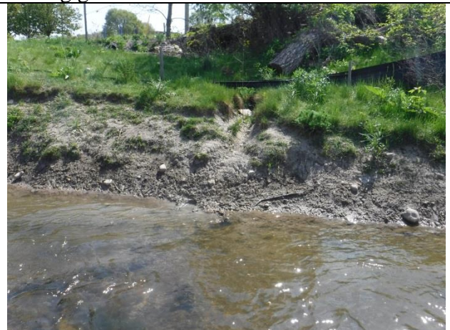
Bank erosion associated with storm sewer outfall
