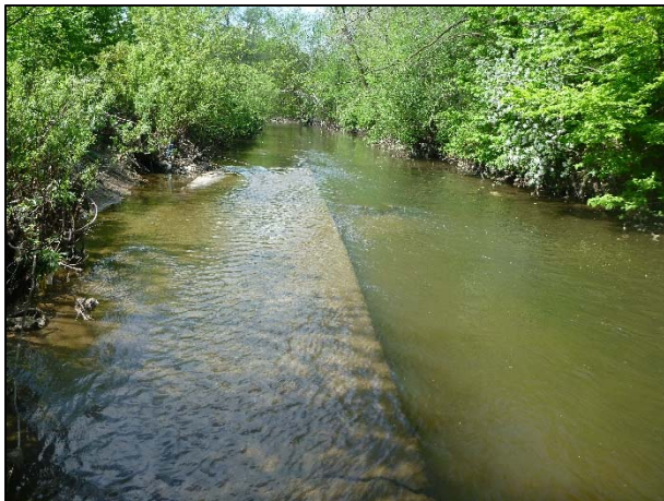
Figure 8-1: Exposed concrete conduit on channel bed at LRL-E5
