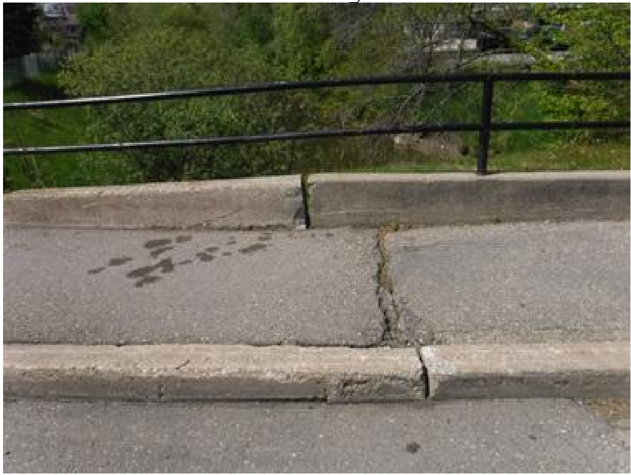
CRACKS IN CURB AND ASPHALT ON BRIDGE DECK
