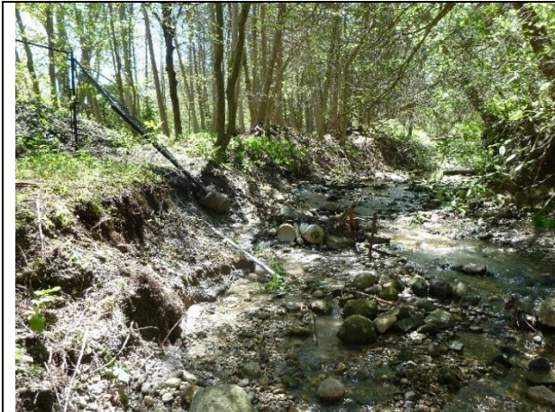
Undermined and leaning fence post
