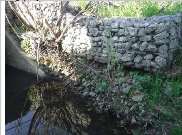
Condition of gabion baskets on right bank
