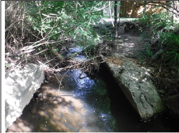
Failing concrete bank treatments may be causing conveyance issues
