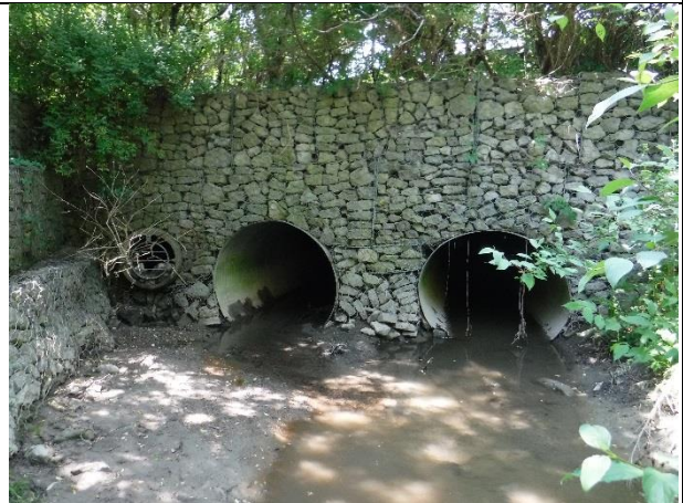
Gabion basket headwall at Columbia Street with lower baskets emptying. Note deformation of culvert on right side of photo.
