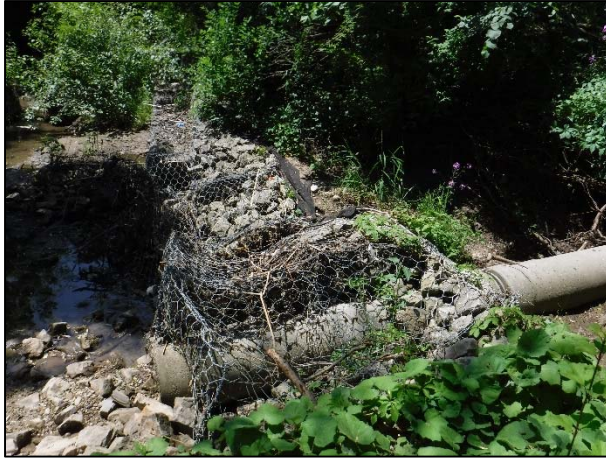
Figure 8-8: Failed gabion basket treatment and exposed storm sewer outfall at CLR-E4
