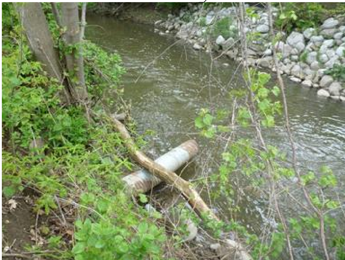
STORM OUTFALL IN POOR REPAIR
