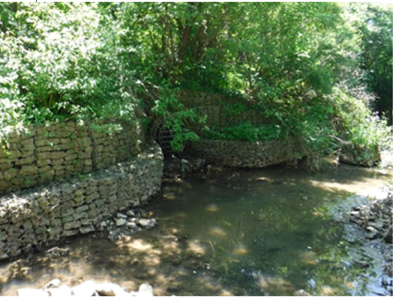
GABIONS AROUND SECOND OUTFALL WITH ENERGY DISSIPATER GABION BLOCK IN CENTRE OF CHANNEL UPSTREAM
