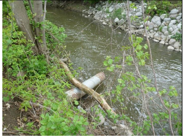
Storm outfall in poor repair
