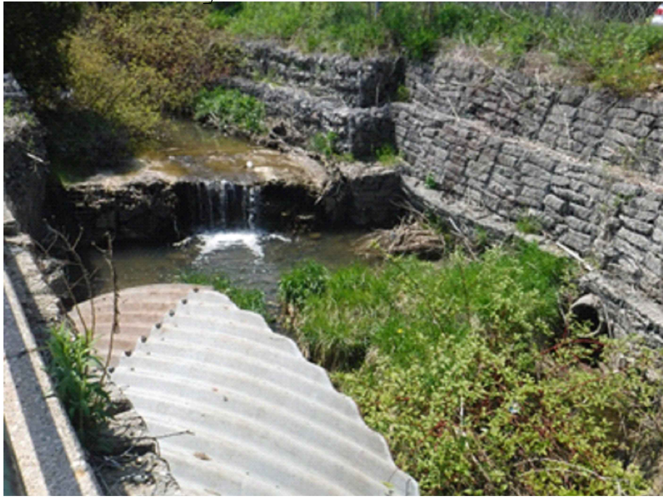
FAILING CONCRETE AND GABION BASKET WEIR ON UPSTREAM SIDE OF ALBERT STREET
