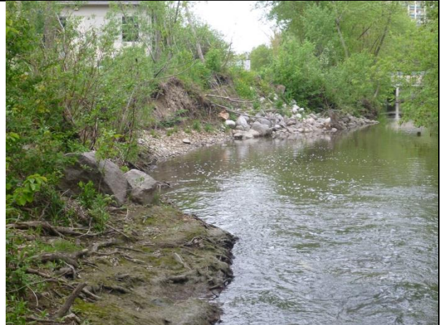
Erosion upstream of roundstone treatment
