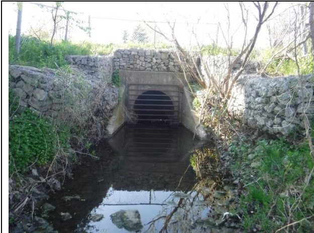
Gabion basket headwalls are slumping and emptying
