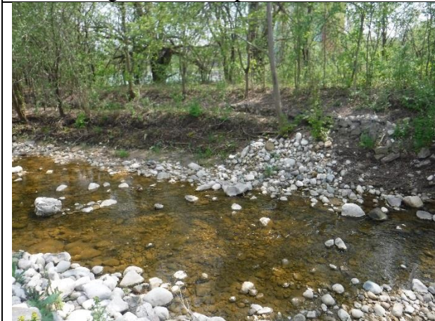
Roundstone bank treatment is failing
