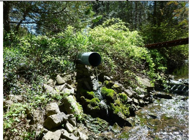
Perched storm sewer outfall
