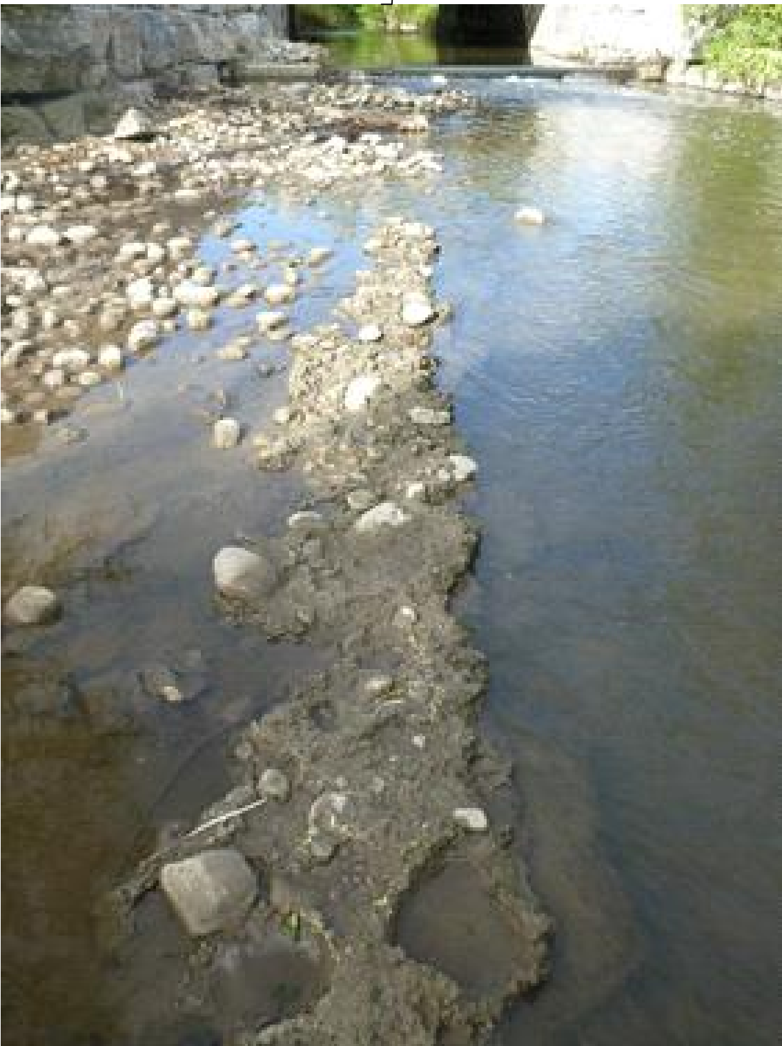
EXPOSED CONCRETE ON BED
