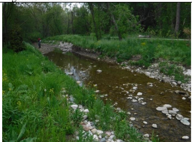
Bank erosion between roundstone treatments with trail in background
