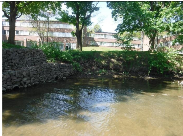
Bank erosion upstream of gabions on right bank
