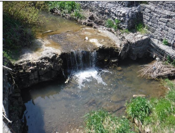
Failing gabion basket weir
