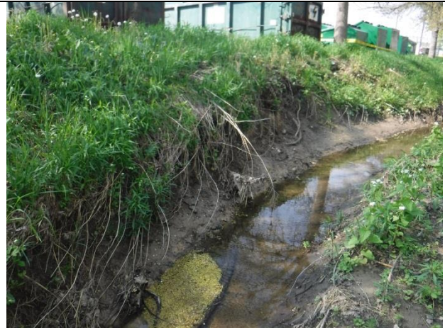
Bank erosion towards parking lot and dumpsters
