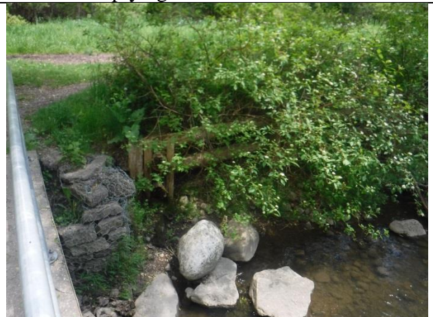
Crib wall in poor condition but vegetation well established
