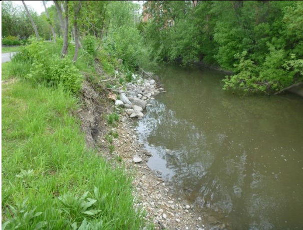
Near vertical bank erosion adjacent to trail
