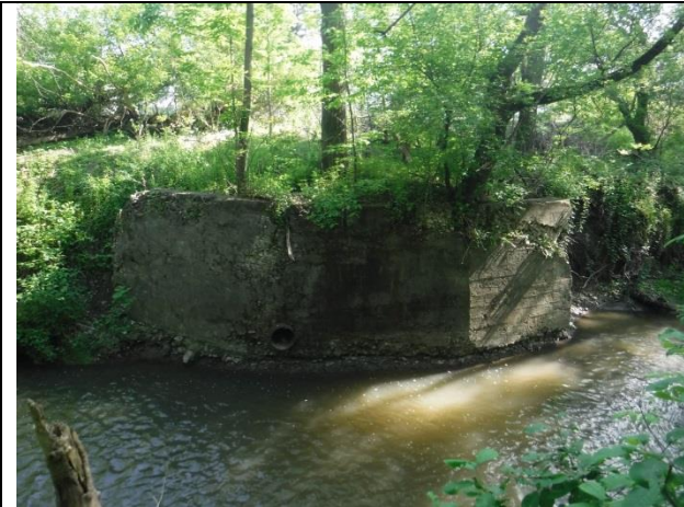
Outflanked old concrete abutment
