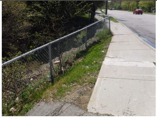
Sidewalk cracked on downstream side of Albert Street
