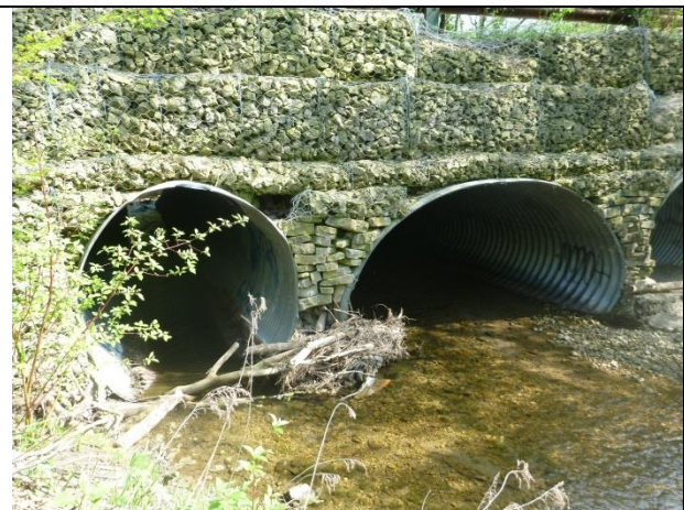
Upstream face of culverts
