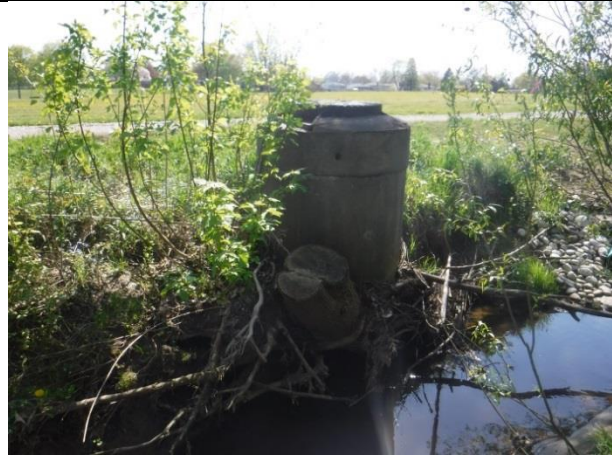
Location 1 – MH with stump of tree at base
