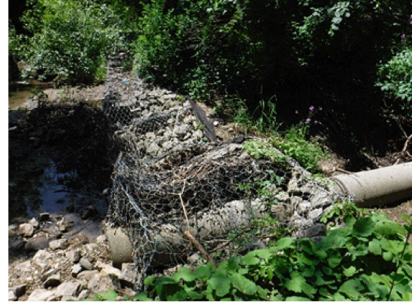
FAILED GABIONS OVER STORM SEWER OUTFALL
