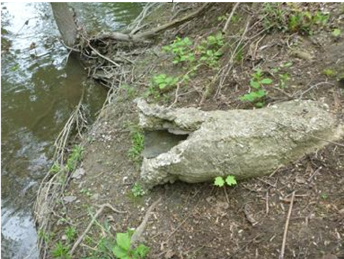
STORM OUTFALL IN POOR REPAIR
