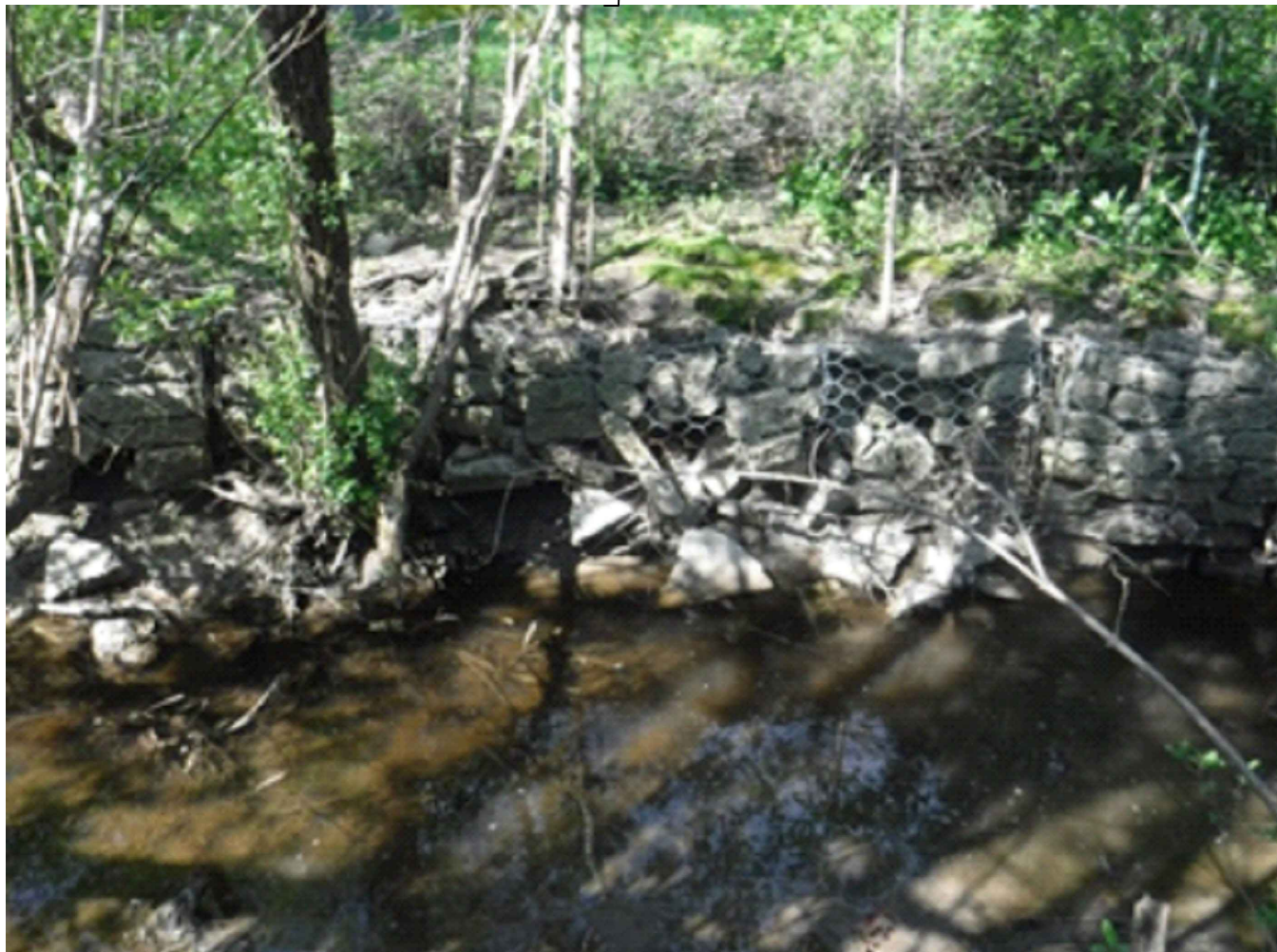
LOCATION 2 - FAILING GABION BASKETS ON LEFT BANK
