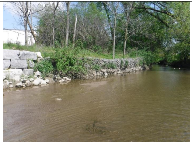
Failing gabions at end of armourstone wall
