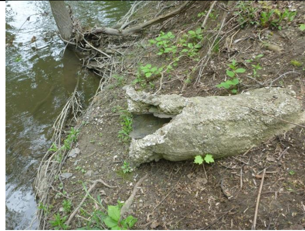
Storm outfall in poor repair
