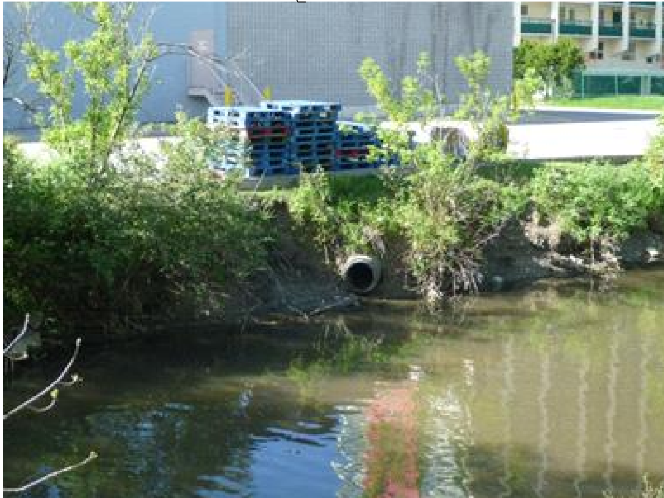
STORM OUTFALL ON ERODED BANK WITH LOADING AREA ABOVE
