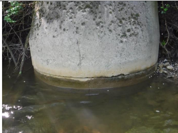
Infiltration may be occurring in joints and cracks in the concrete
