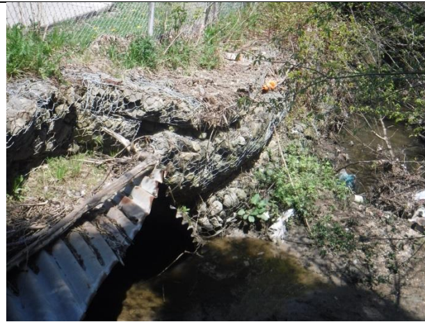
Detail of condition of collapsing culvert on downstream side of Albert Street
