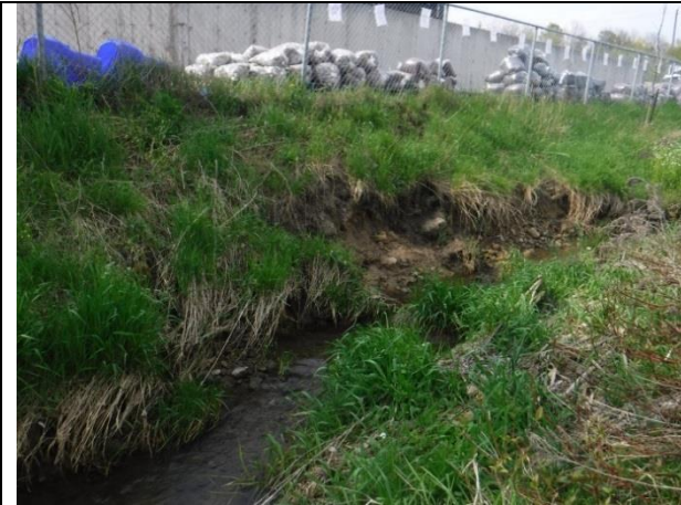
Bank erosion and slumping adjacent to garden centre lot
