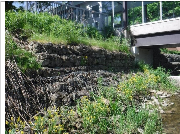
Emptying gabion baskets downstream of crossing for University of Waterloo residence (REV)
