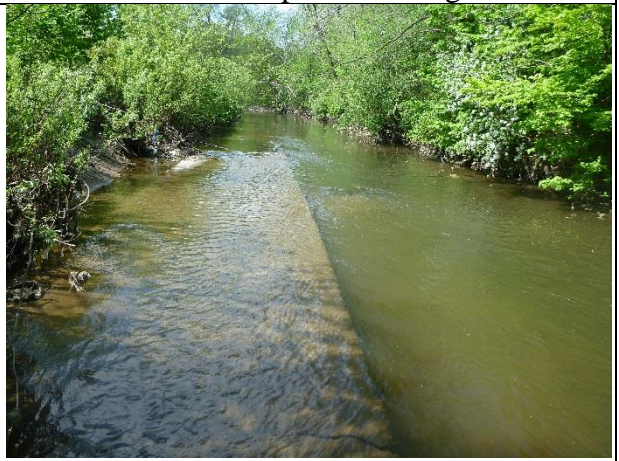
Exposed concrete on channel bed
