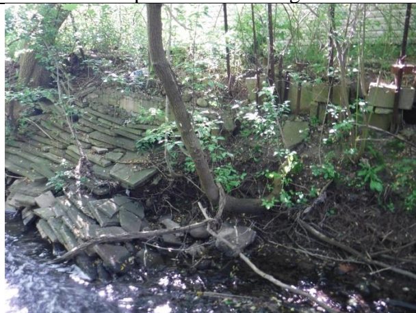
Failing privately constructed concrete slab and concrete block bank treatments
