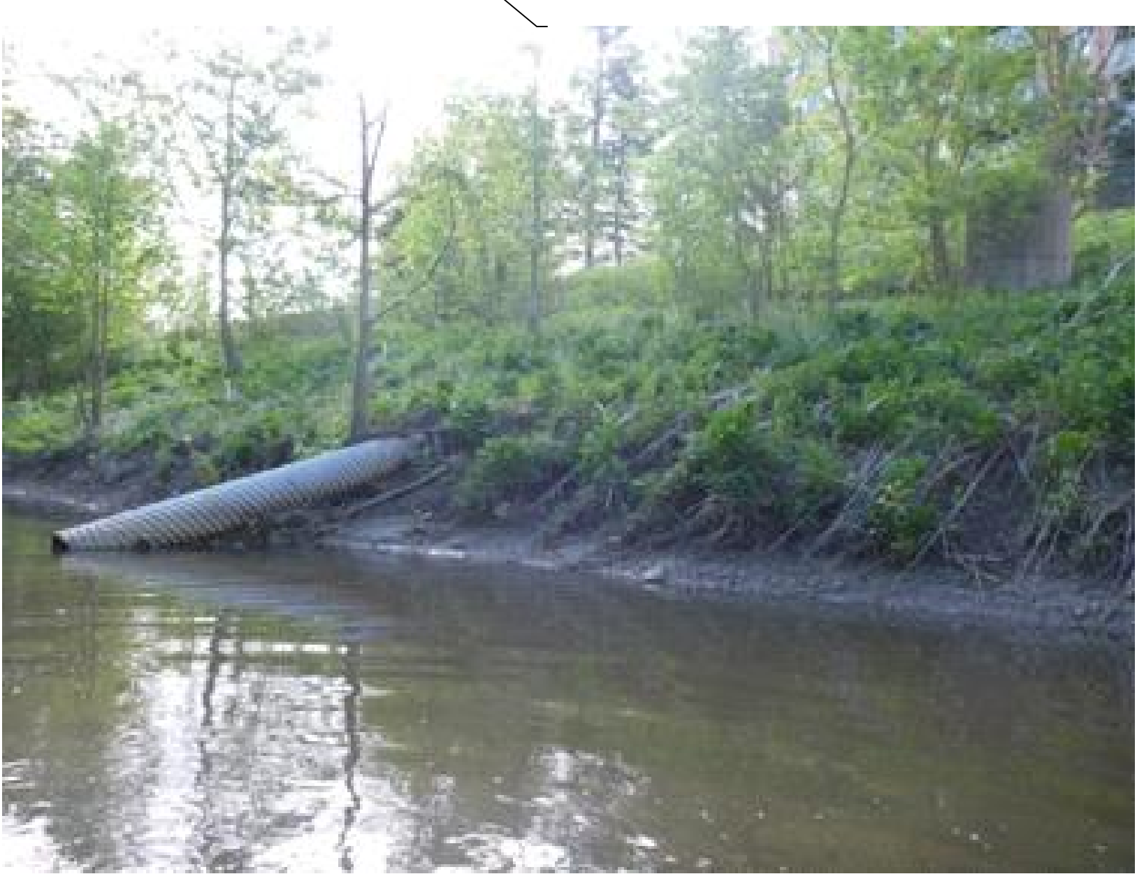
NEAR VERTICAL BANK EROSION IN FRONT OF MH. FAILING PRIVATE OUTFALL.
