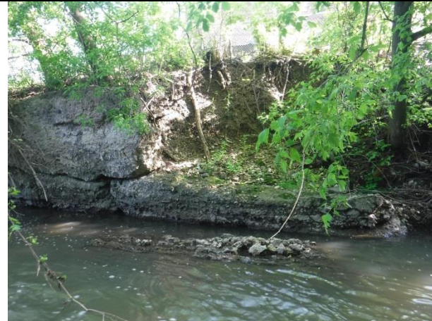
Outflanked downstream end of concrete wall
