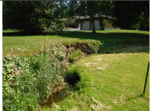
Eroded and slumping banks
