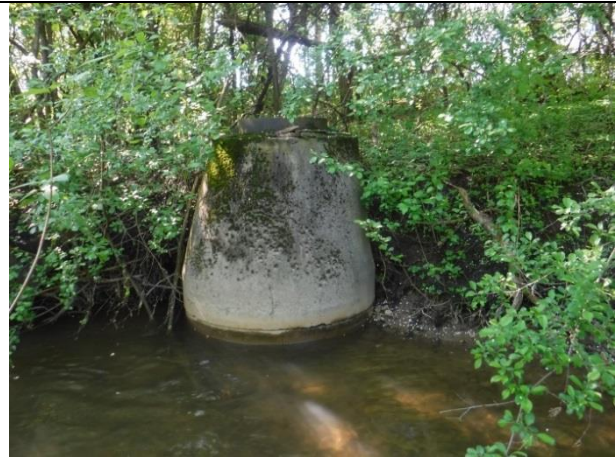
Approximately half the circumference of the MH is exposed
