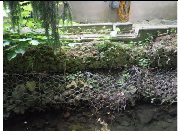
Failing gabion baskets
