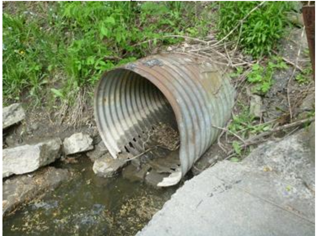
STORM OUTFALL IN POOR CONDITION
