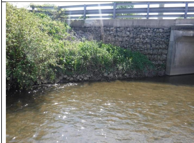
Failing gabion toe on right bank
