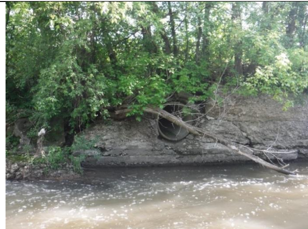
Storm sewer outfall in concrete wall
