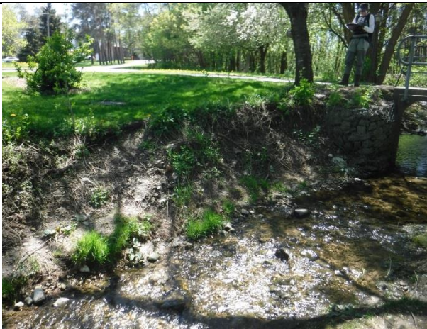
Steep, eroded bank with MH in grass at top
