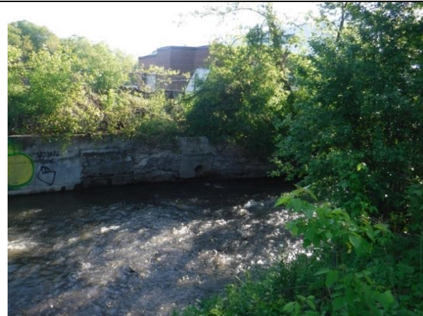
Leaning concrete wall with storm sewer outfall
