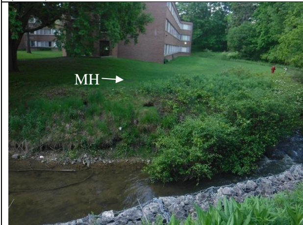
Sanitary sewer MH behind eroding bank
