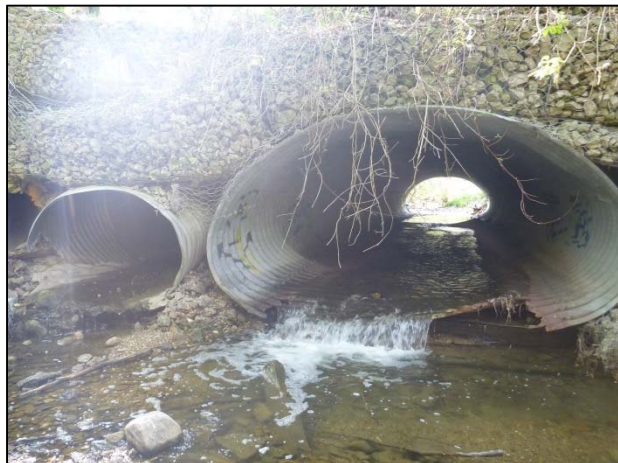
Figure 8-4: Failing, undermined culverts on downstream side of Forwell Creek Road crossing at FRW-E2
