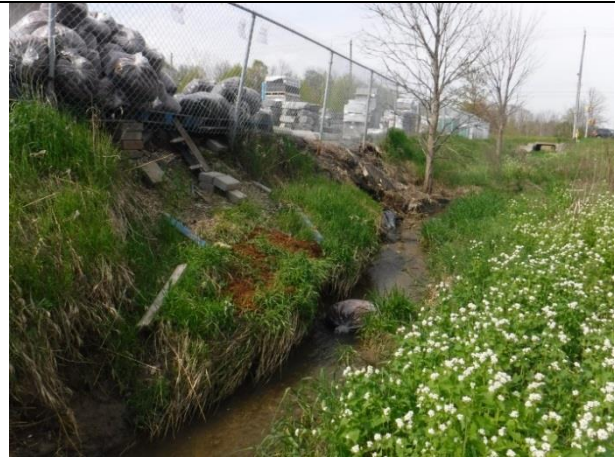
Undermining of fence
