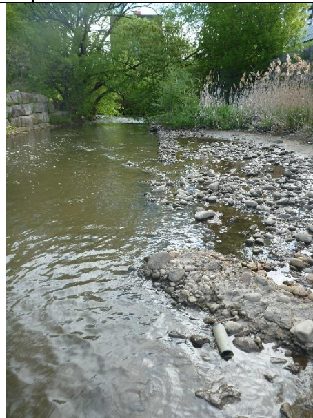
Exposed concrete on bed
