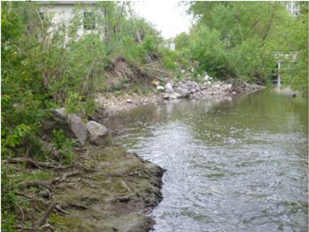
EROSION UPSTREAM OF ROUNDSTONE TREATMENT
