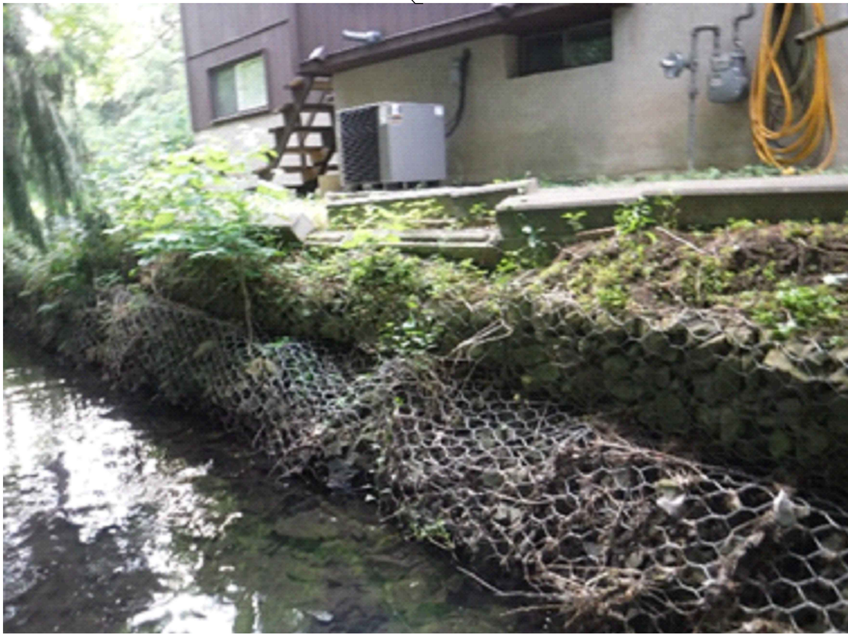
FAILING GABION BASKETS
