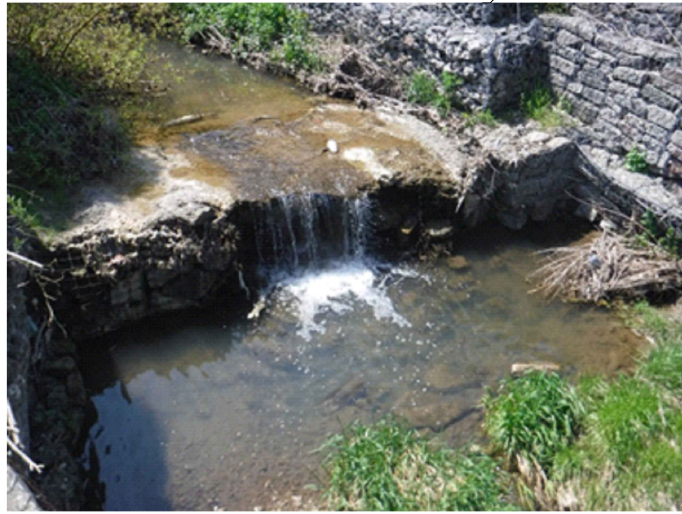
FAILING GABION BASKET WEIR
