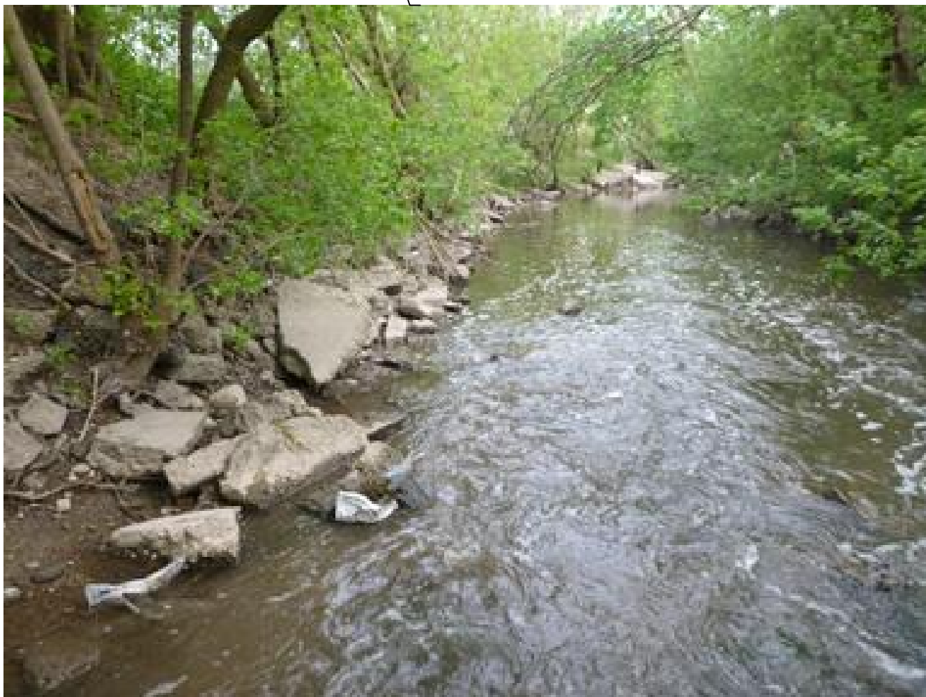
CONCRETE DEBRIS ON TOE OF BANK
