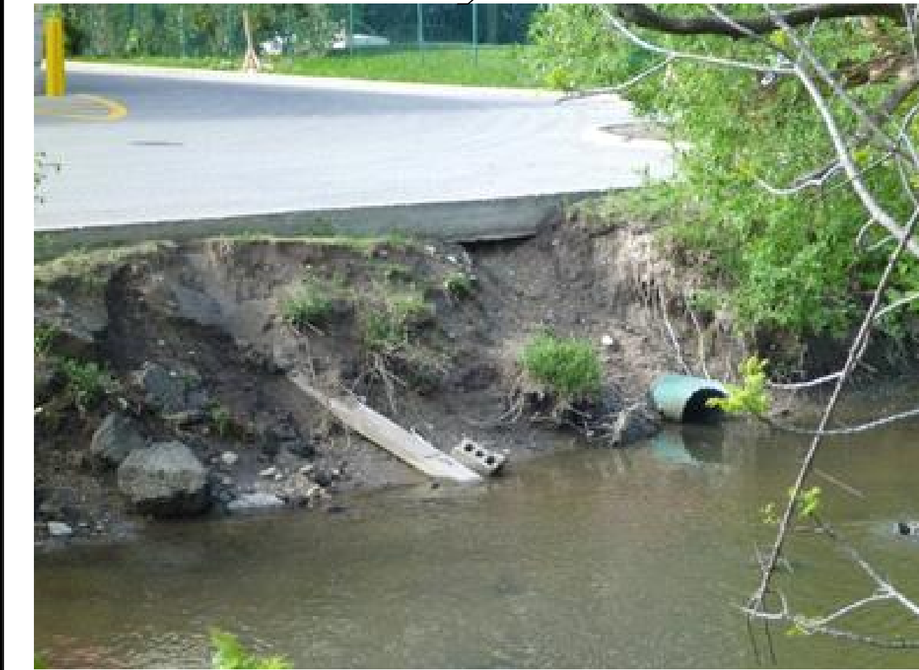
UNDERMINING OF LOADING AREA PAVEMENT
