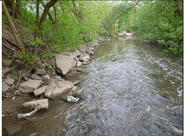
Concrete debris on toe of bank
