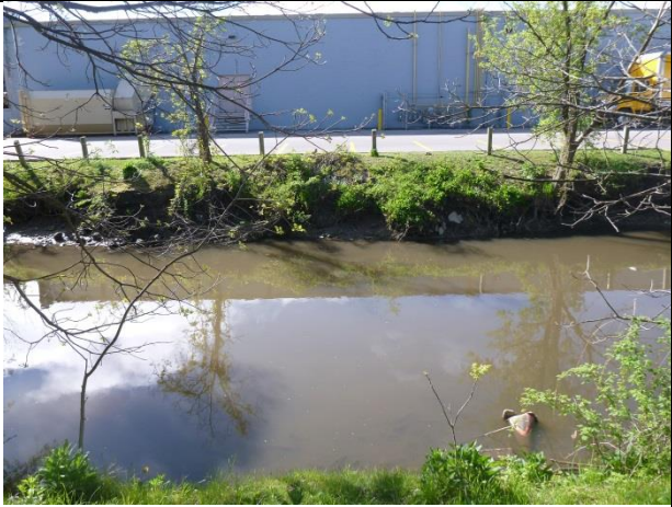
Bank erosion adjacent to paved loading area
