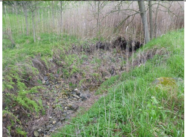
Bank erosion near storm sewer outfall
