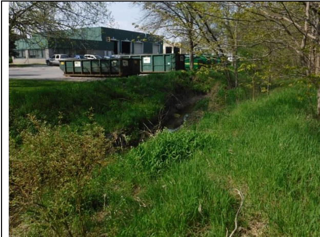
Bank erosion towards parking lot and dumpsters
