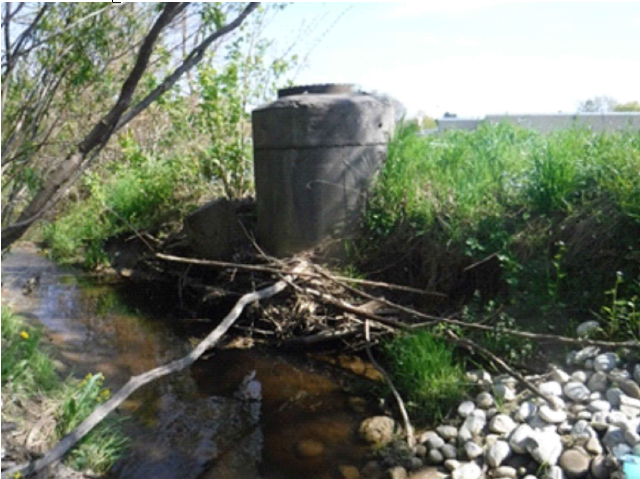
LOCATION 1 - SCoured BANK IMMEDIATELY UPSTREAM OF MH
