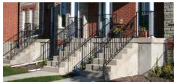
Concrete poured-in-place steps are favoured over pre-cast steps (Waterloo).
