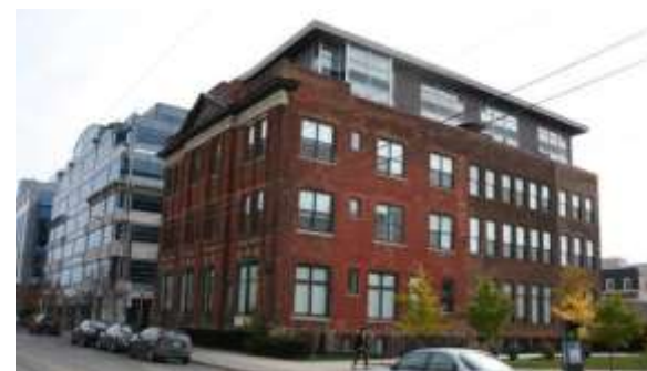
A compatible development may include contrasting elements which distinguishes new additions from the existing structure (Toronto).
