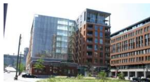
A curtain wall system creates a transparent façade from the surrounding park, and also, maximizes views into the park (Montréal).
