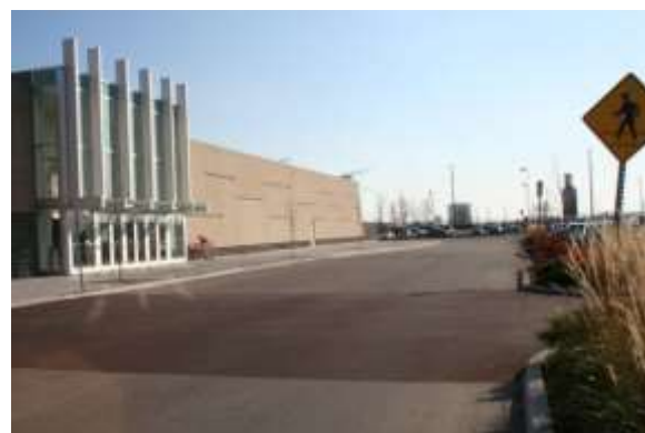
For select locations, a raised platform provides an effective traffic calming feature (Waterloo).
