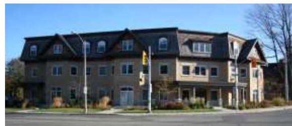
Direct and safe pedestrian access is provided when buildings are located adjacent to the street (Kitchener).
