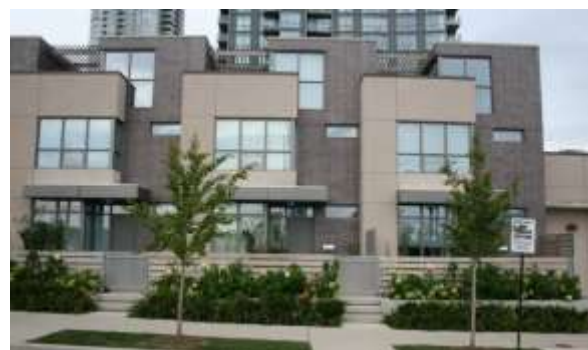
The quality of building is enhanced through brick walls, strong over-door canopies and large windows (Toronto).
