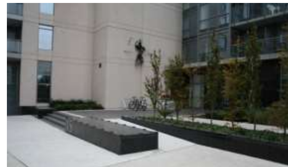
Barrier free access should be provided at primary building entrances and architecturally integrated with the building and site design (Toronto).
