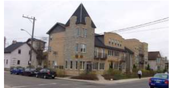
Articulated facades create interest along the street and can be used to create a focal point (Waterloo).
