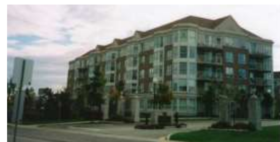
An interesting roofline is created through a pitched roof with gable dormers (Waterloo).
