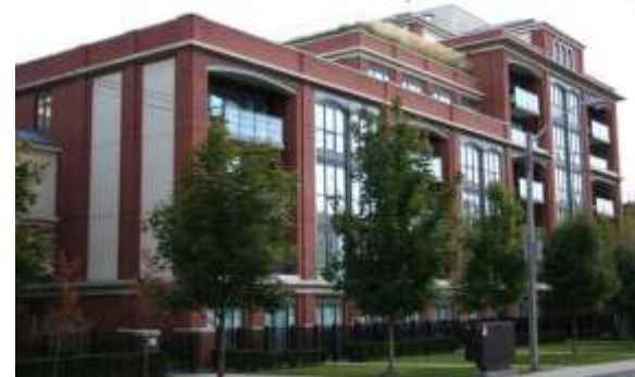
Privacy is improved when new development incorporates recessed or partially recessed balconies (Toronto).
