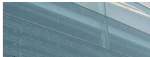
Glass etching provides opportunity to integrate public art into building facades (National Ballet School, Toronto).
