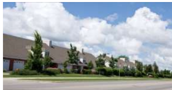
Landscape berms provides an effective buffer from cars and noise along busy roads (Kitchener).
