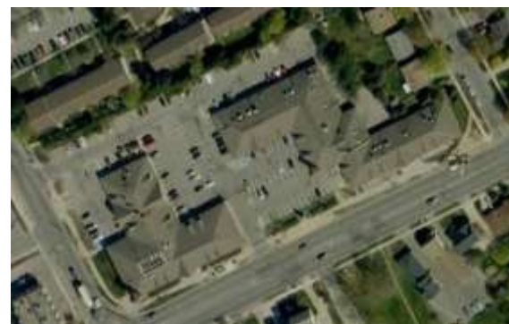
The impact of parking areas is reduced when parking is located in side and rear yards (Waterloo).
