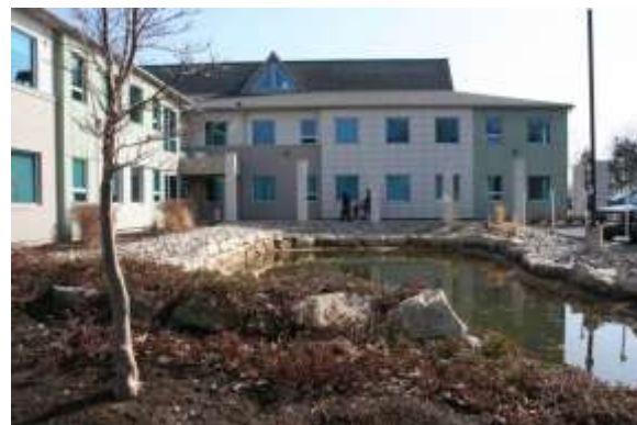
On-site water quantity and quality is improved through integrated stormwater management pond (Kitchener).
