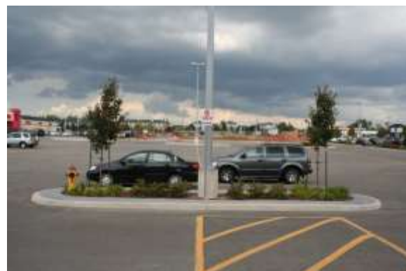
Traffic islands provide ideal locations for fire route signage and fire hydrant locations (Waterloo).
