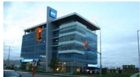
Layered massing and a cantilevered roof structure create interest to relatively simple building shape (Brampton).
