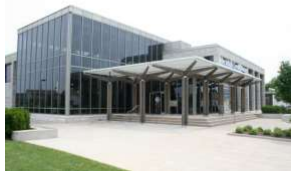
An architecturally designed shelter creates an interesting and comfortable outdoor amenity space (Niagara-on-the-lake).
