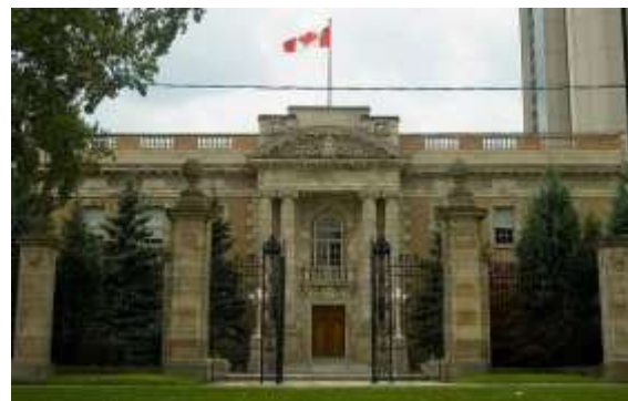
The Sunlife building is a prominent landmark in the City and designated as a heritage building (Waterloo).
