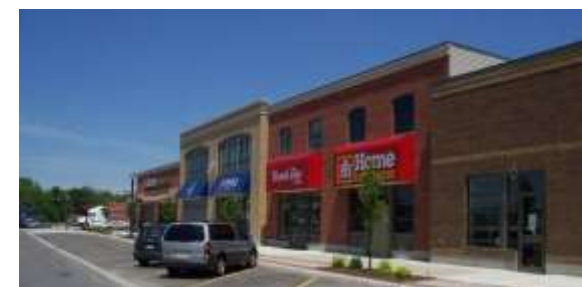
Long commercial façades are softened through window treatment, cornices and vertical bays (Kitchener).
