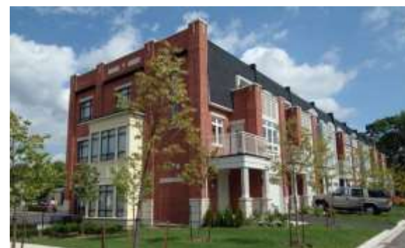
A consistent level of architecture is create when the design of side and rear elevations complement the primary façade (Mississauga).
