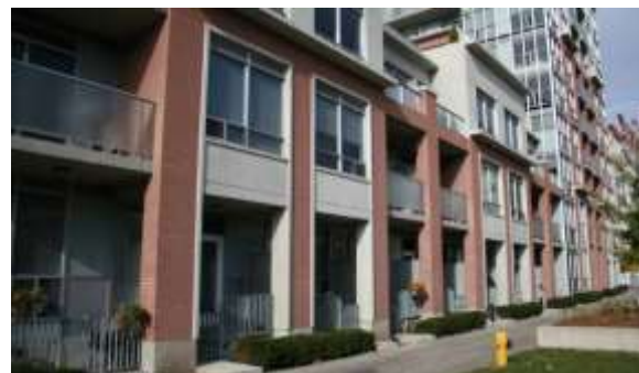
High quality materials include brick, concrete, cornices, spandrel glazing and curtain wall systems (Toronto).
