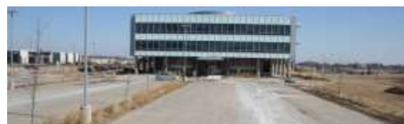
A bio swale provides opportunity to introduce sustainable design into site development (Waterloo).
