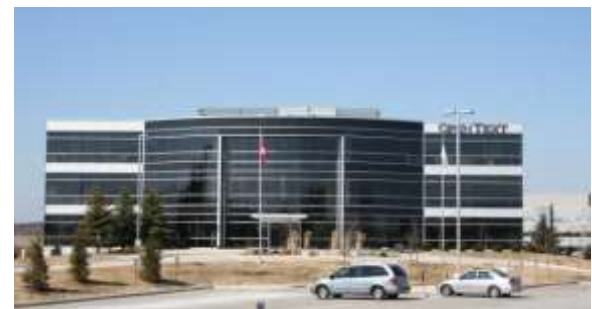
Louvered screens effectively hides roof top mechanical equipment from public view (Waterloo).
