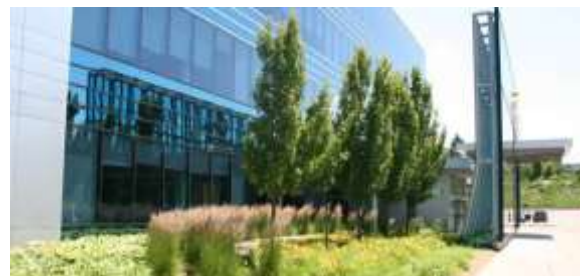
Visual interest is increased through variation in height, form and material (Waterloo).
