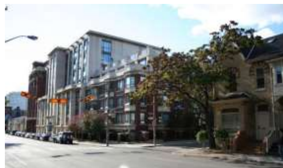
A stepped building form results in less wind and shadow impacts to surrounding properties (Toronto).
