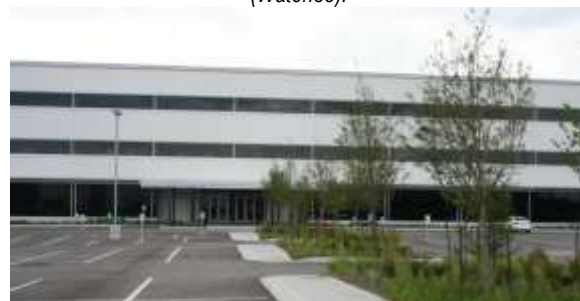
Urban heat island effect and the scale of large parking areas is reduced through landscaped islands and walkways (Waterloo).
