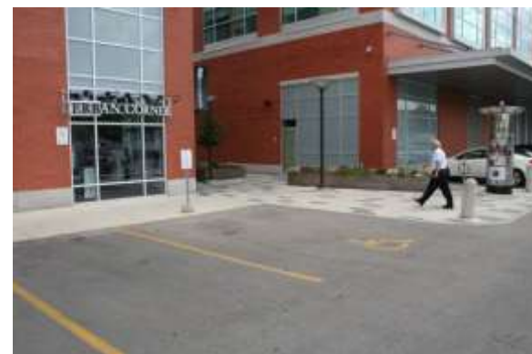
The City standard for barrier free parking is the “flush curb” design which provides a smooth transition in grade between the abutting sidewalk and barrier-free parking space (Waterloo).
