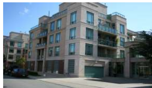
Efficient access is provided when the parking garage entrance is located close to the street (Toronto).
