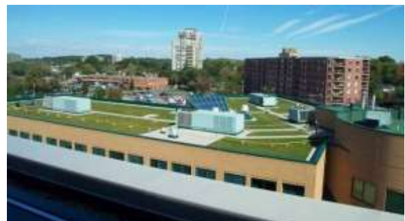
Green roof technology helps reduce urban heat island effect (Waterloo).
