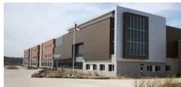
Vertical elements, layered massing and variation in material and colour help reduce the scale of large buildings (Waterloo).
