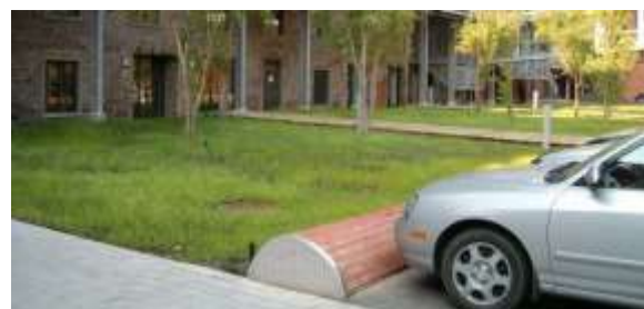
Creative details, such as an industrial curb stop, can add interest in a development and contribute to a development theme (Montréal)
