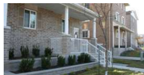
Prominent entrance features require larger decorative columns (Waterloo).
