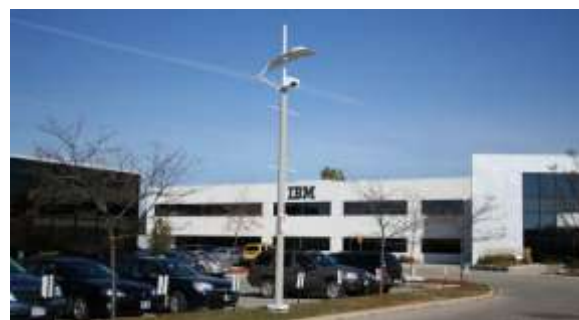
Major site entrances can be enhanced through architectural light fixtures (Waterloo).
