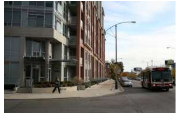
Accessibility and convenience is improved when building entrances are located close to the transit stop (Toronto).
