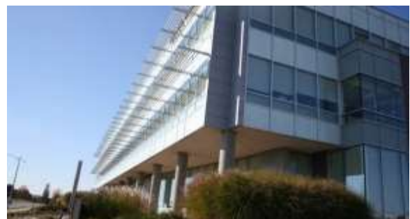
Shadows and increased expression can be achieved through architectural design details such as screens, spandrel panels and box bay windows (Waterloo).
