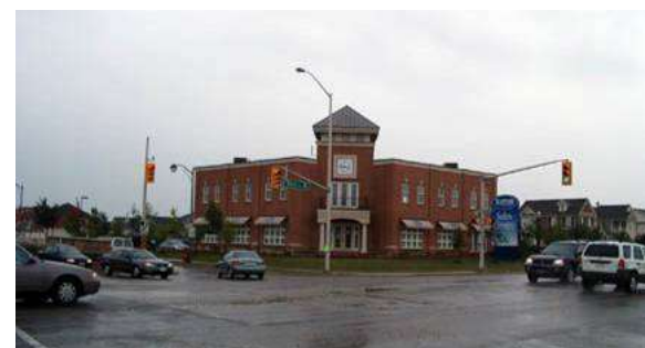
Vertical elements provide an interesting view at major intersections (Milton).
