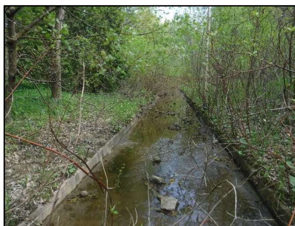
Figure 3.9.2: Hardened Channel on Forwell Creek
