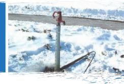
Rink hydrants are designed and installed to be self-draining, allowing them to operate in colder temperatures without freezing.
